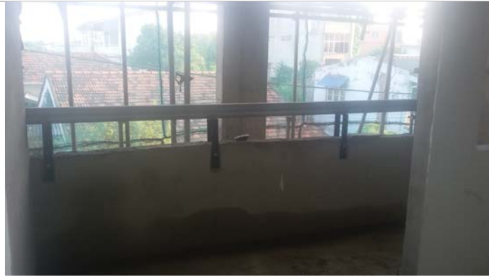
Fixing Balcony Railing at 1 st Floor
