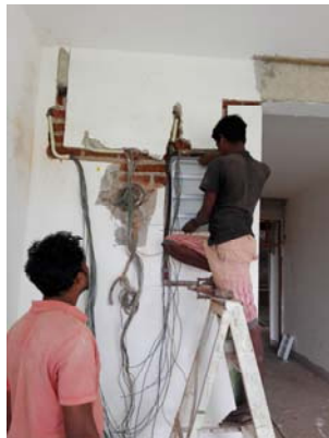
Electrical Work at 2 nd Floor
