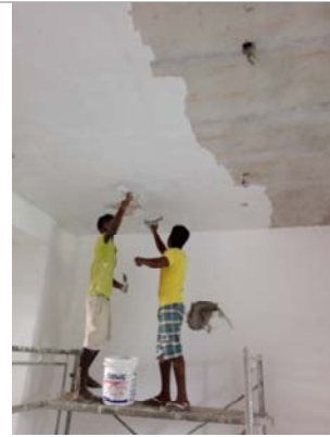
Putty Application Work at 2nd Floor
