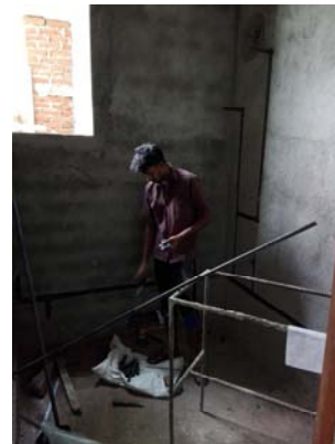
Plumbing for Water Supply line at 3 rd Floor
