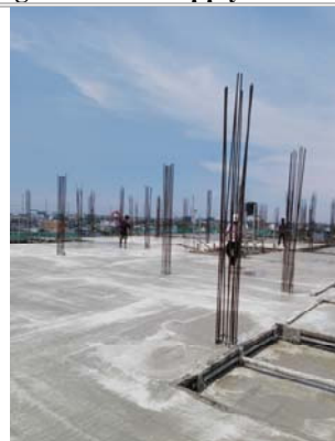
7 th Floor Slab
