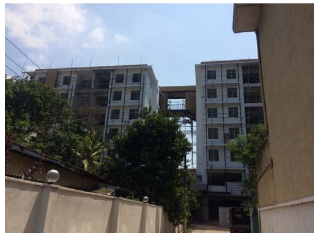
External painting work in progress
