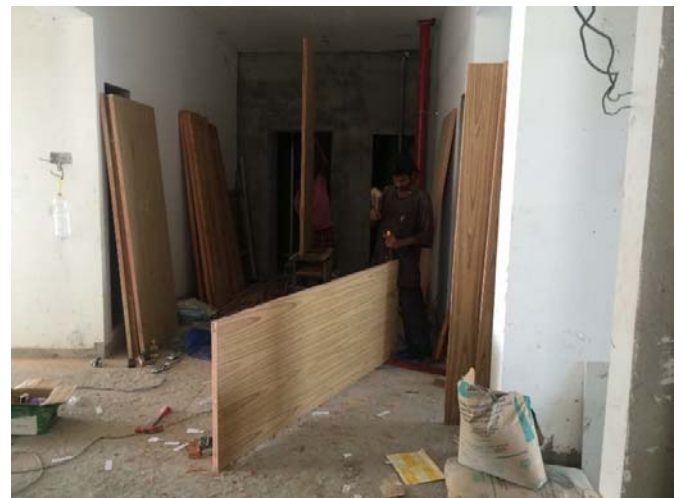
Door fixing work in progress
