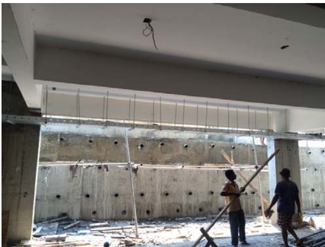
Parking area painting work in progress
