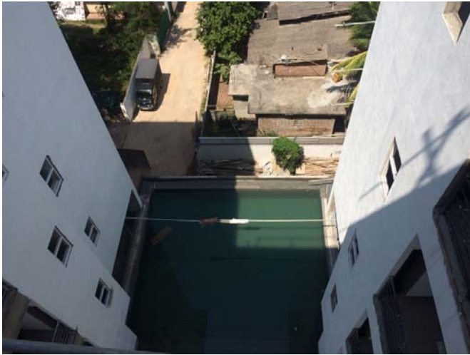
Pool deck tiling work in progress
