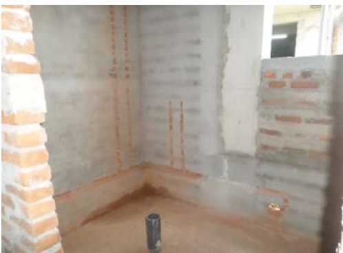
Tower 02 - 1 st Floor Plumbing Work on Progress
