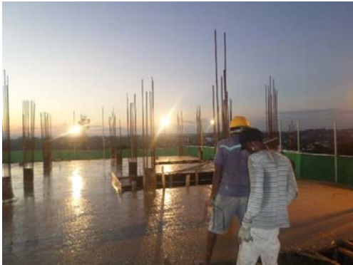
Tower 02 – 5 th Floor Casted on 30/03/16
