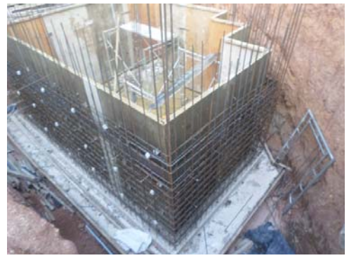
Watersump Walls R/F & F/W on Progress
