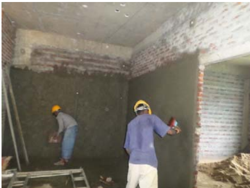
Tower 02 – 1 st Floor Plastering on Progress
