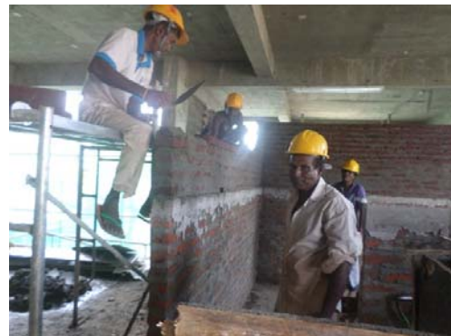
Tower 02 – 2 nd Floor Brickwork on Progress
