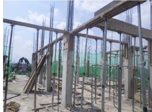
Tower 01 - 5 th Floor Slab F/W on Progress
