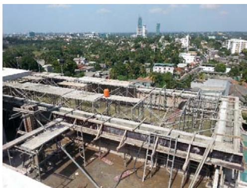
Tower 01 – Swimming Pool Structural works completed
