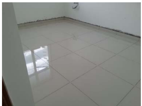
Tower 01 – 2 nd Floor Tiling work on progress
