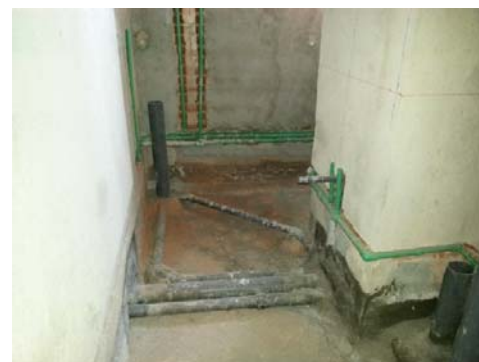
Tower 01 – 6 th floor Plumbing work on progress
