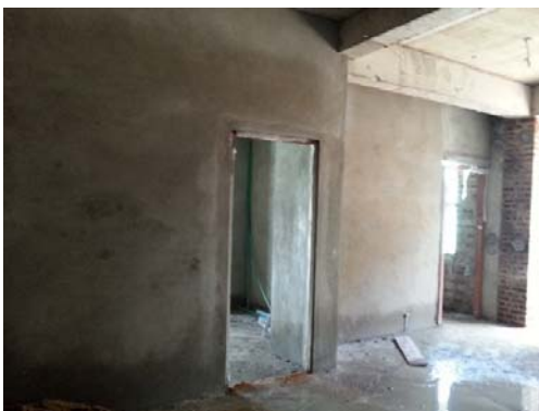
Tower 01 – 7 th floor Plastering on progress
