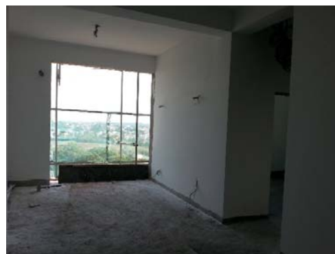
Tower 02 – 6 th floor Painting work on progress
