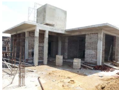
Tower 01 – Roof terrace Masonry works
