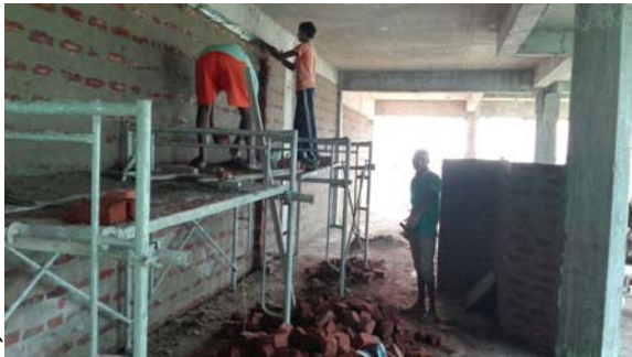
Brick Work- 8 th Floor
