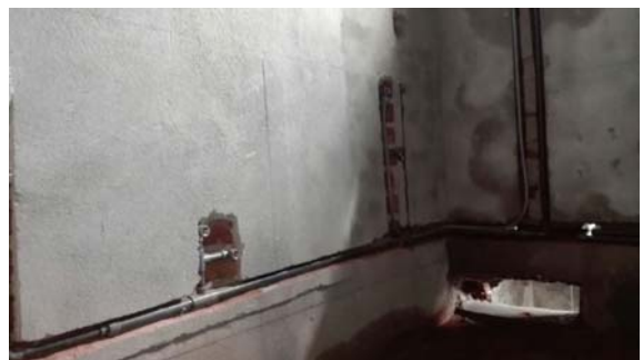
Plumbing work- 4 th Floor
