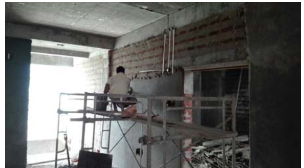
Internal Plastering- 7 th Floor
