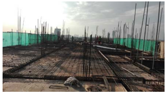
Reinforcement Work- Slab 10 th Floor (G4 to G10)
