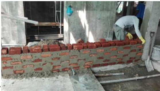
Brick Work- 9 th Floor
