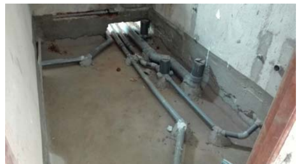
Plumbing work- 3 rd Floor
