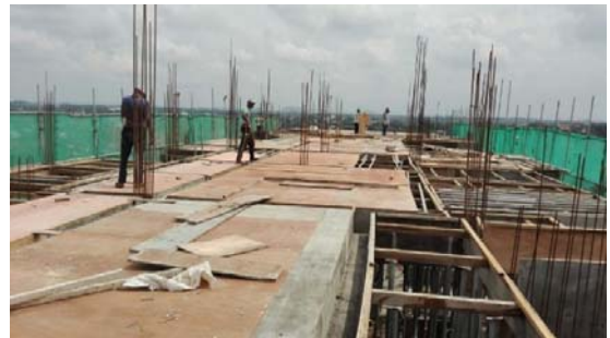
Form Work- Slab 11 th Floor (G4 to G16)
