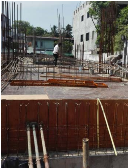
Ground floor work on progress
