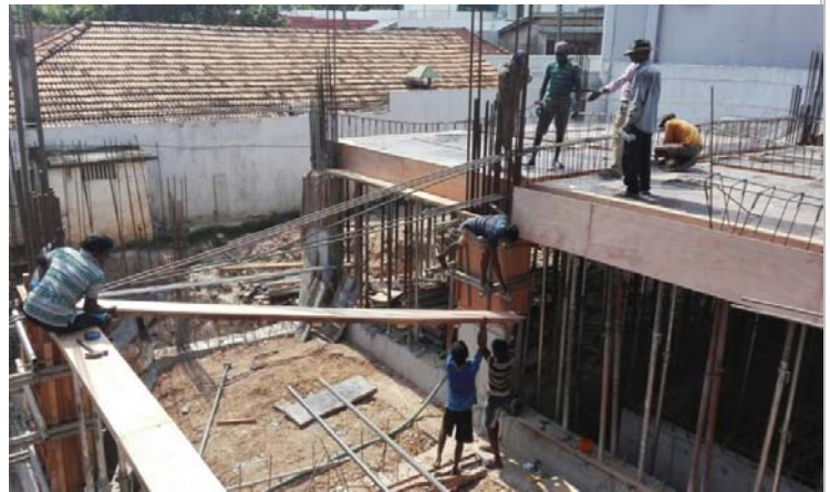
Ground floor work on progress
