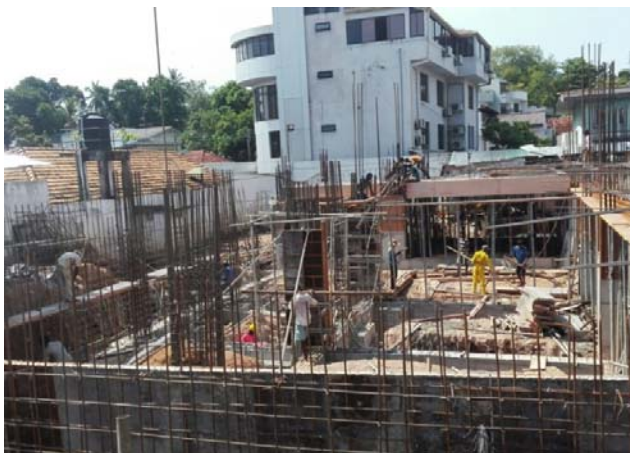
Retain wall work on progress
