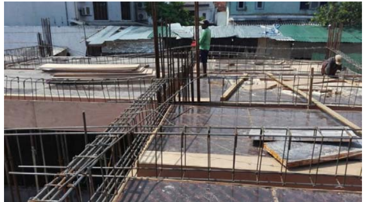
Ground floor work on progress
