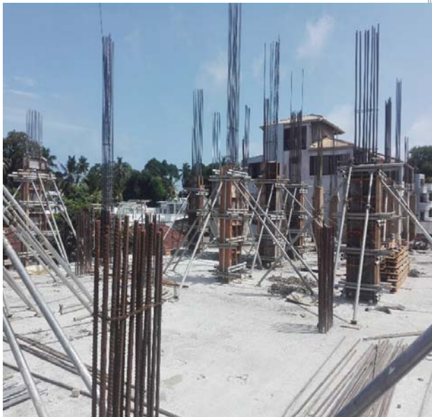
1 st floor column formwork on progress
