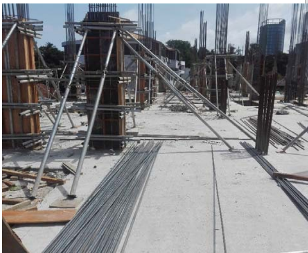
1 st floor beam reinforcement work
