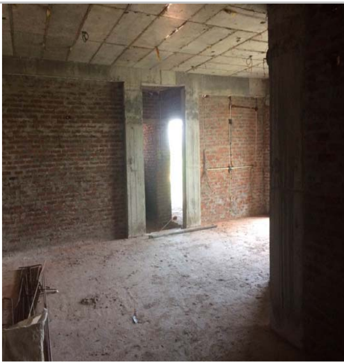
5 th floor brick work
