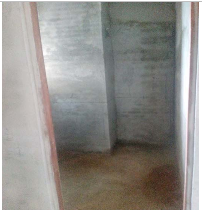
4 th floor plaster work
