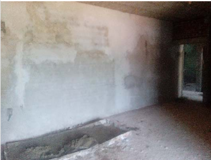
5 th Floor plaster work
