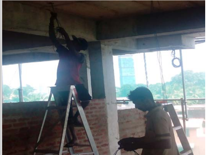
5 th Floor Electrical wiring
