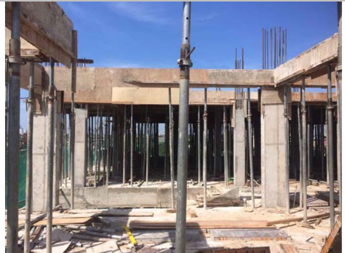
8 th floor slab formwork
