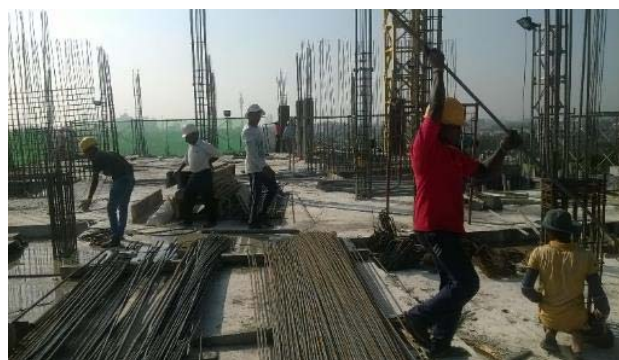
6 th FLOOR COLUMNS
