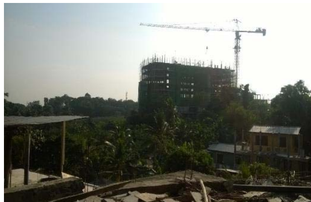
SITE VIEW FROM VILLAGE END
