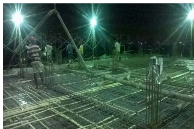
CONCRETING 6 th FLOOR SLAB
