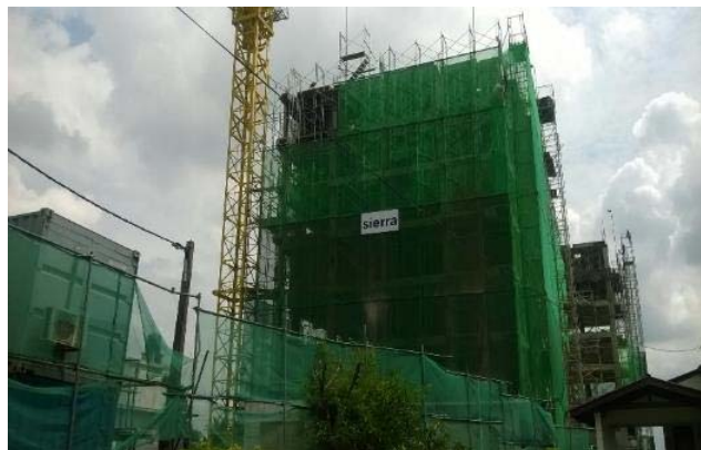
SITE FRONT VIEW
