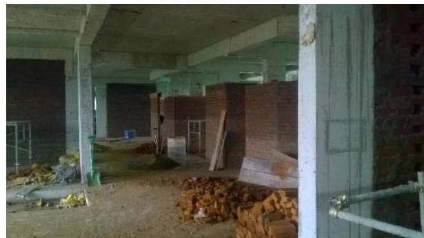
BRICK WORKS-3 rd FLOOR
