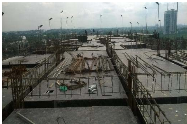
WORKING FOR 7 th FLOOR SLAB
