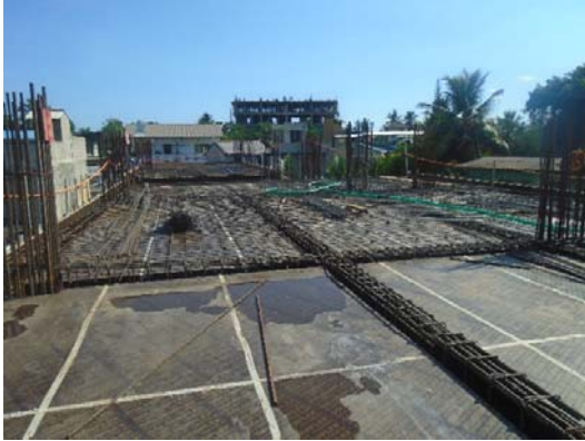
Slab r/f work
