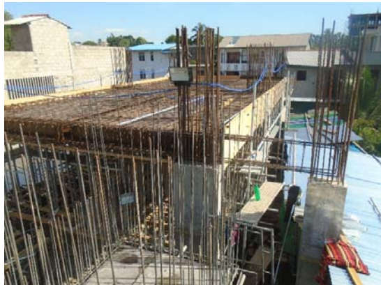
Slab r/f work
