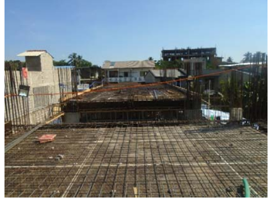
Slab r/f work
