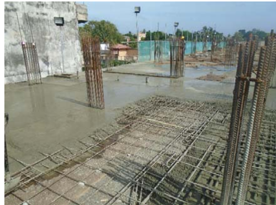
FF Slab concreting on 15/06/2016
