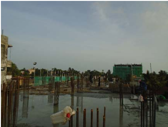
FF Slab concreting on 15/06/2016
