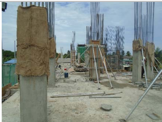
FF-SF Column work
