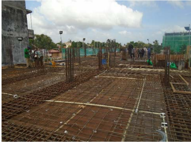
FF Slab ready for concrete
