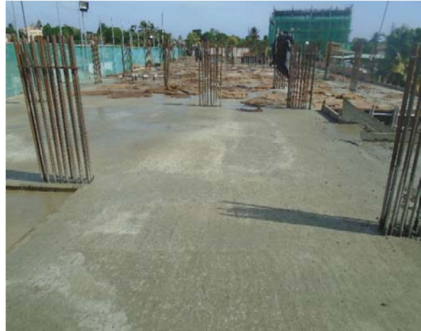
FF Slab concreting on 15/06/2016
