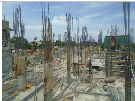
FF-SF Column work
