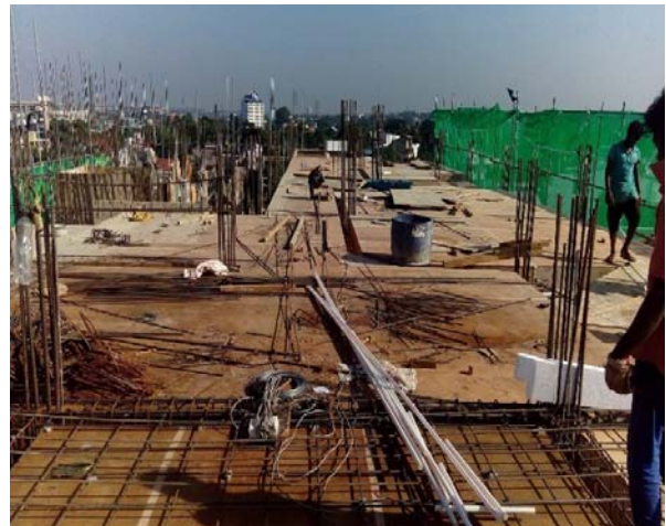
Seventh Floor Slab formwork work in progress
