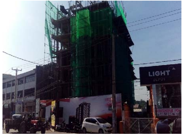
Front view of the building
