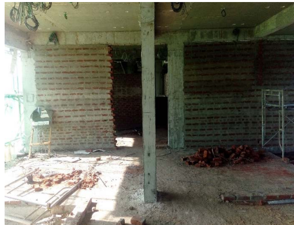
Fourth Floor Brick work in progress
