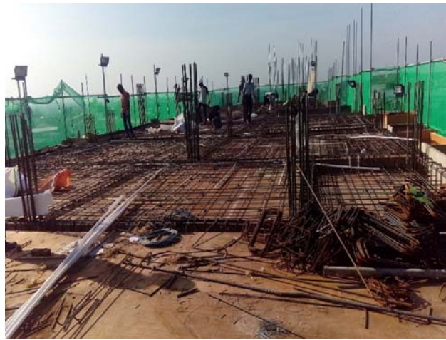
Seventh Floor Slab reinforcement work in progress
