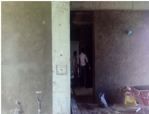
Fourth Floor Plastering work in progress
