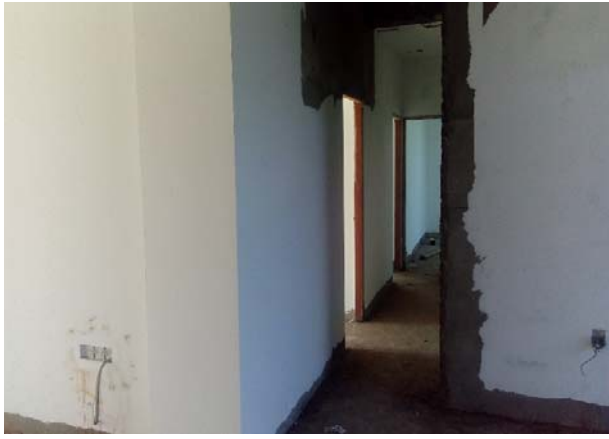
First Floor Putty work in progress
