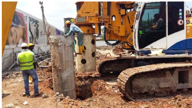
Placing the Pile Casing
