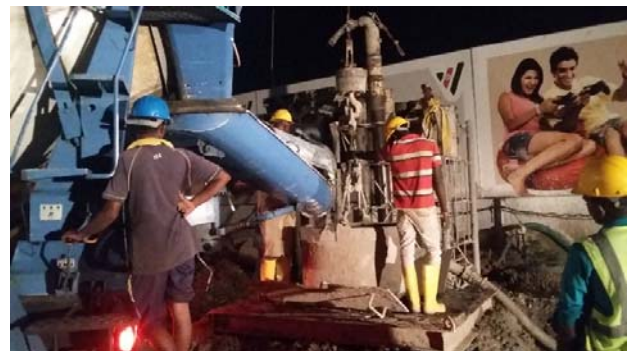
Pile Concreting works
