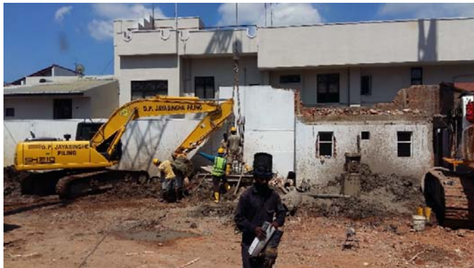
Site Cleaning Works
