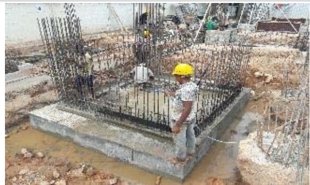
LIFT 01 BASE CURING
