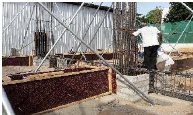
PLINTH BEAMS F/W IN PROGRESS
