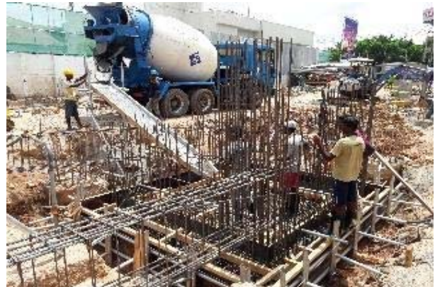
LIFT 01 BASE CASTING
