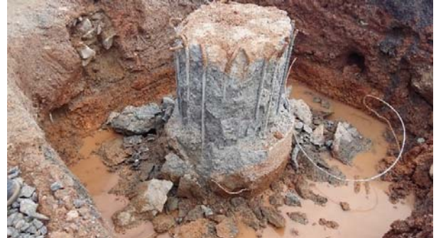
PILE BREAKING FOR FOUNDATION WORK
