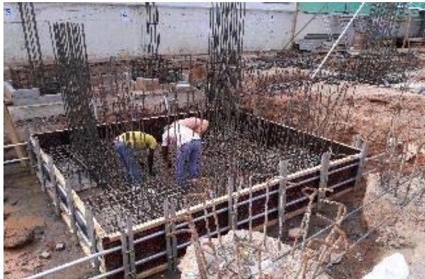
LIFT 01 BASE REINFORCEMENT WORK
