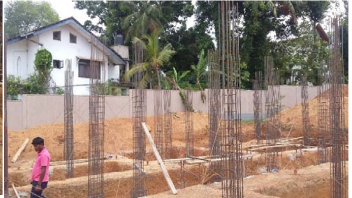
Rebar work in Progress
