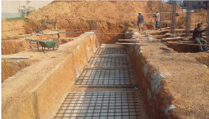
Rebar work in Progress
