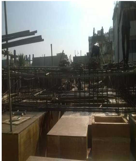
Figure 1 - Re bar work on 1 st floor slab
