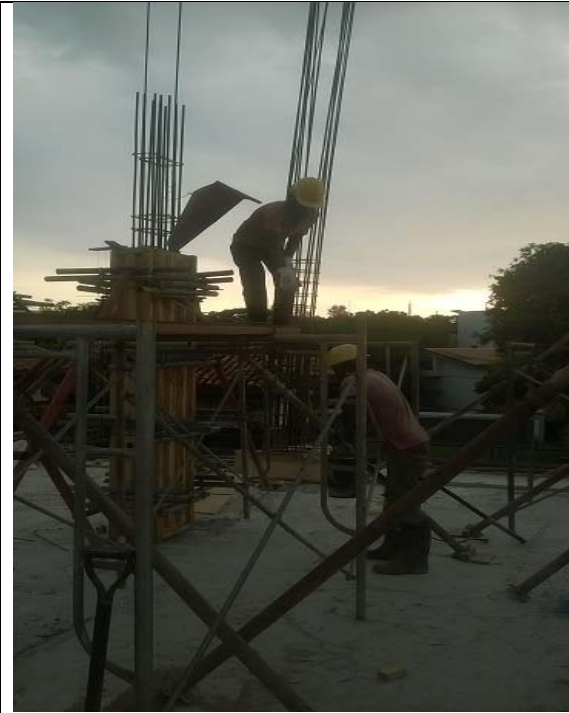
Figure 5- 1 st floor column concreting
