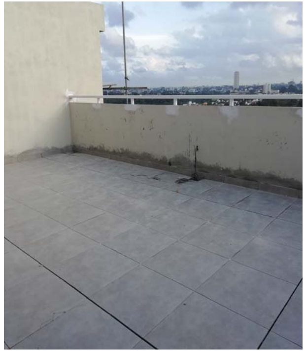
Figure 6 – Roof Terrace Tiling
