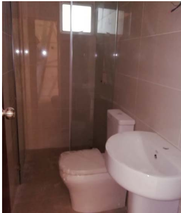
Figure 1- Bath Room Fittings Fixing at 4 th Floor
