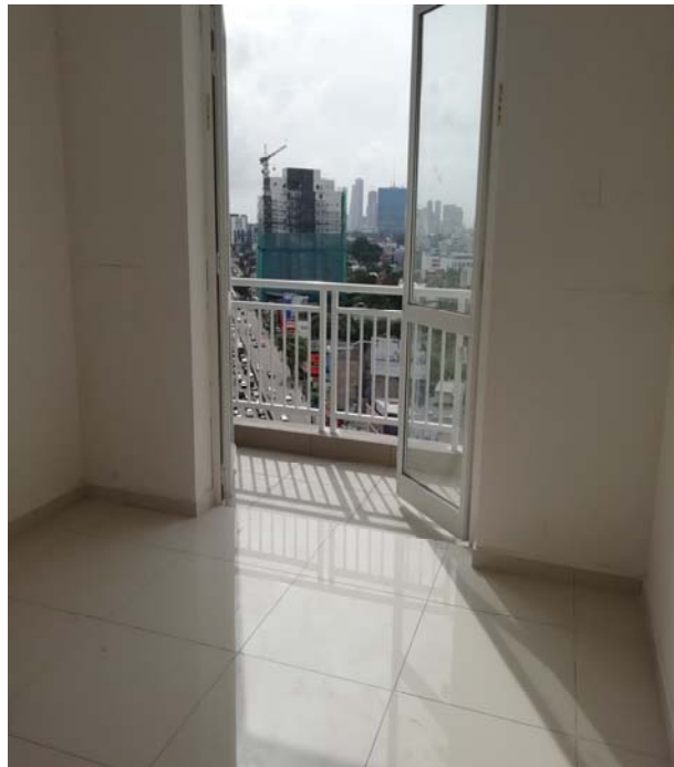
Figure 3 - Aluminum Installation and Balcony Rail Painting at 10 th Floor
