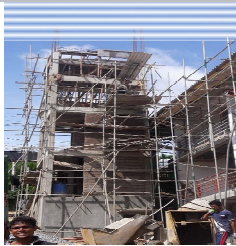
WATER TANK 4 TH FLOOR SLAB FORM WORK OVERALL PROGRESS – 65%
