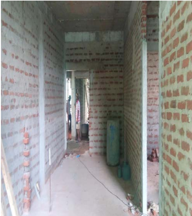
1 st Floor brick work
