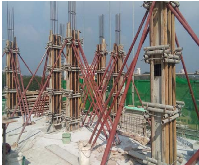
Columns up to 5 th floor
