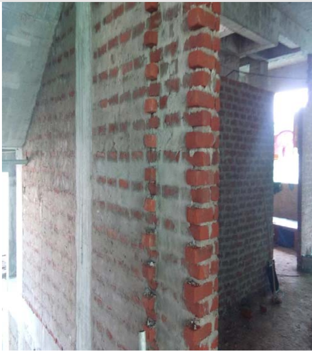
2nd floor brick work
