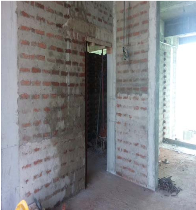
3 rd Floor brick work
