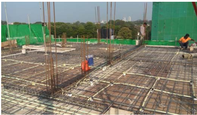
5 th floor slab
