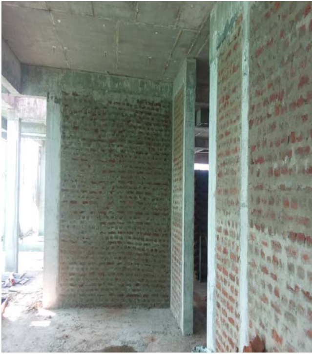
4 th floor brick work
