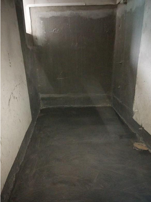
TOILET WATER PROOFING WORK
