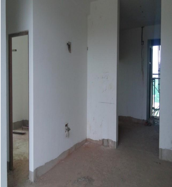
INTERNAL PUTTY WORK
