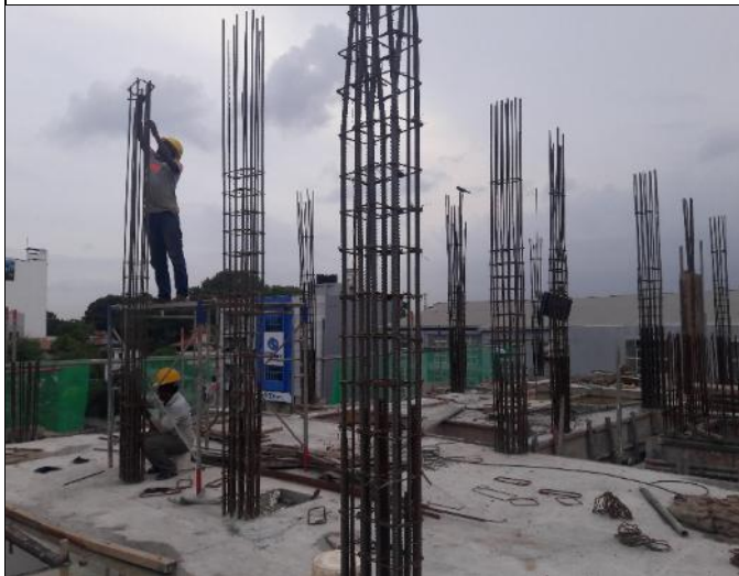
Figure 3.3- 5 th floor column R/F
