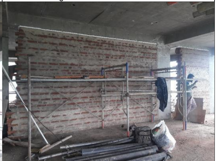
Figure 3.6-1 st floor Brick works
