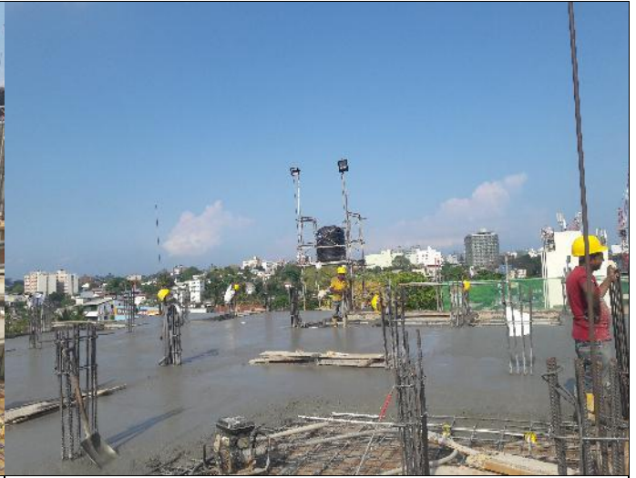
Figure 3.8 – 5 th floor Slab Casting
