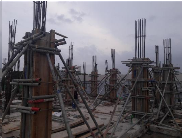
Figure 3.4- 5 th floor column F/W
