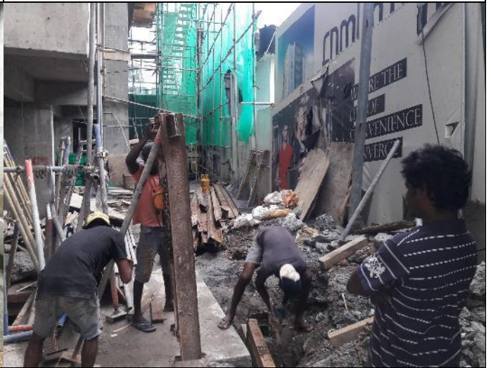
Figure 3.10-Shorine removing
