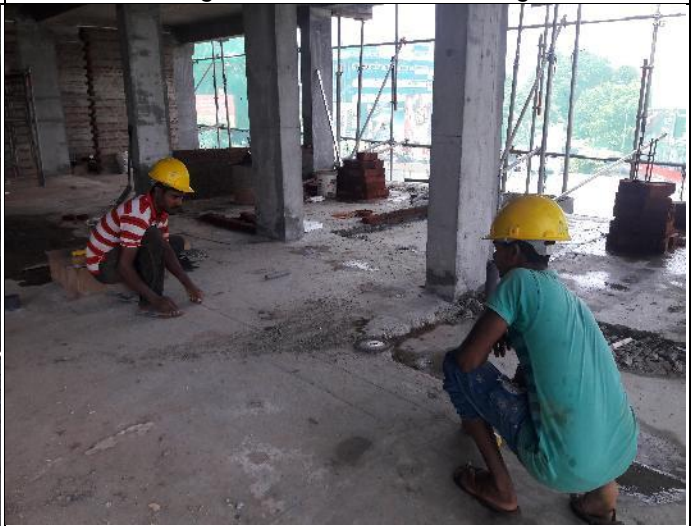
Figure 3.12-Settingout for brick works
