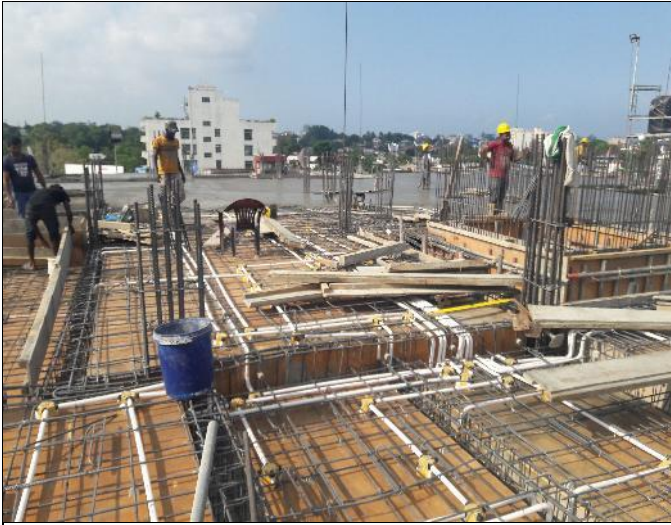
Figure 3.7- 5 th floor Slab F/W
