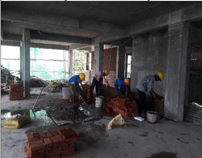
Figure 3.11- Brick works at 2 nd floor
