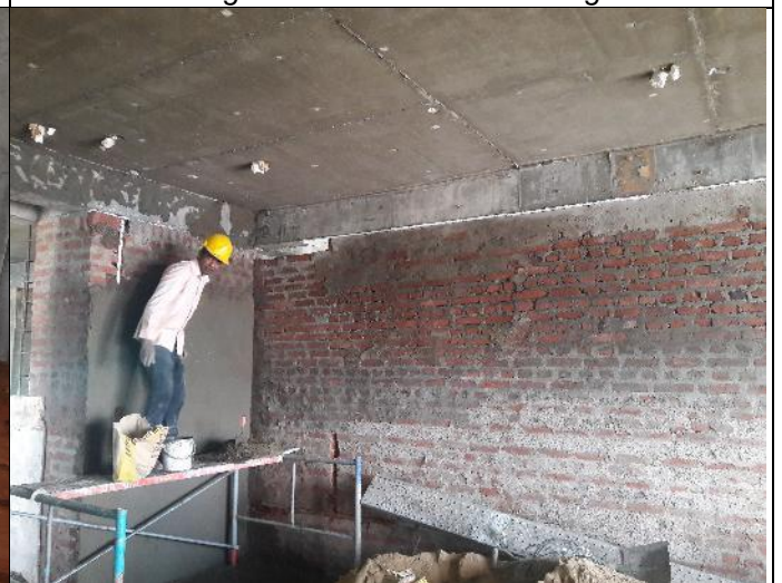
Figure 3.6-3 rd floor plastering
