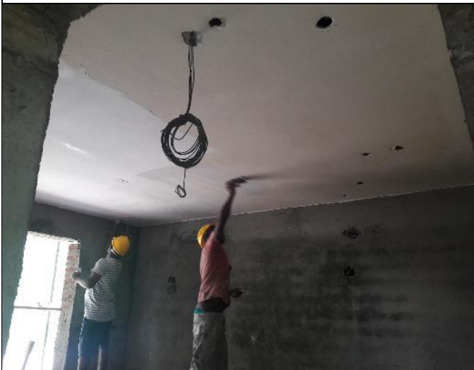
Figure 3.9- 2 nd floor putty works
