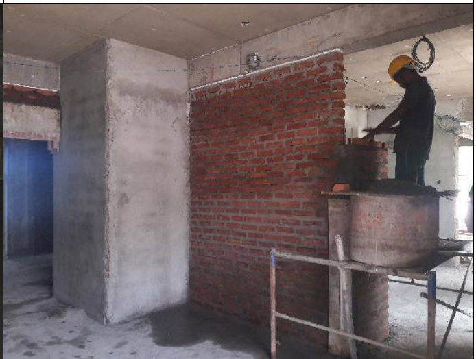
Figure 3.10-2 nd floor Brick works
