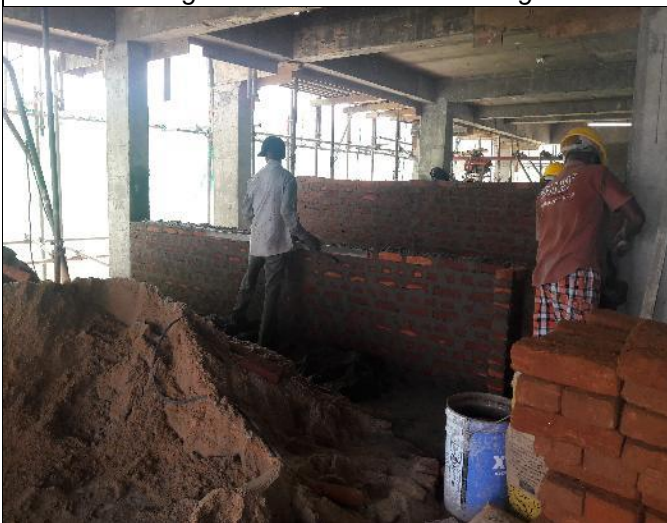
Figure 3.5-3 rd floor Brick works
