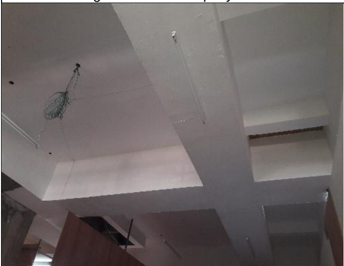
Figure 3.11- 1 st floor putty works
