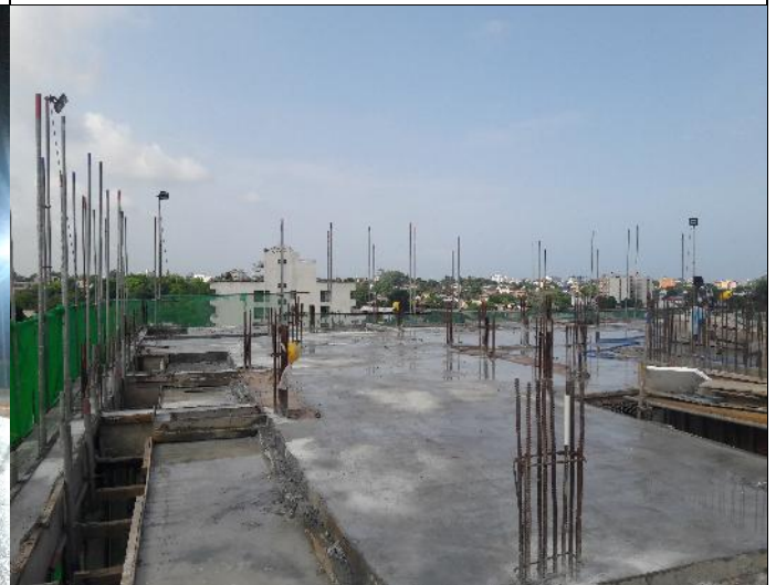
Figure 3.4- 6 th floor slab curing
