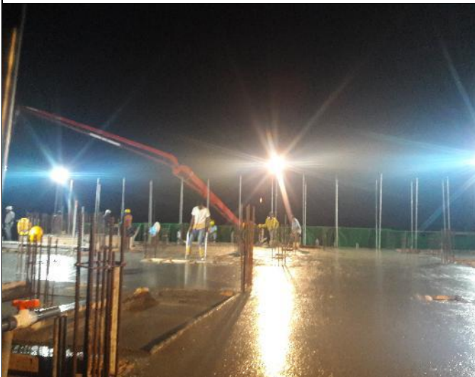
Figure 3.3- 6 th floor slab casting
