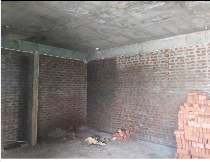
Figure 3.7- 4 th floor Brick works
