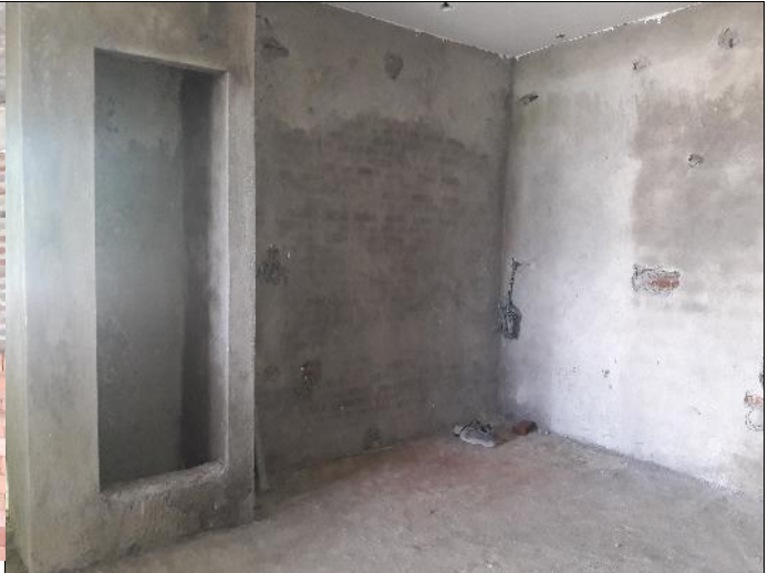
Figure 3.8 – 2 nd floor plastering
