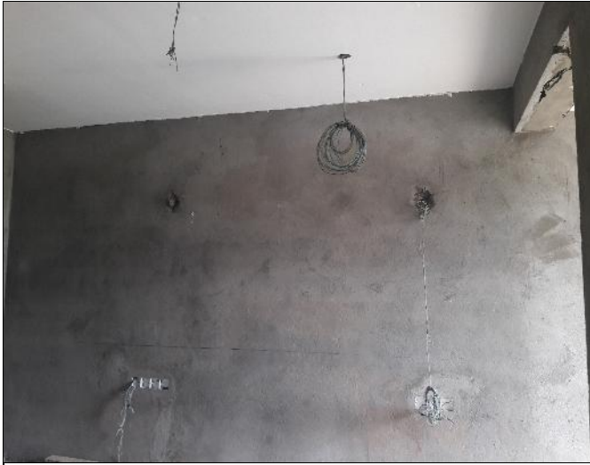
Figure 3.7- 2 nd floor electrical works
