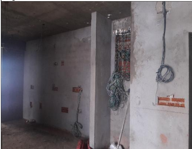
Figure 3.5-3 rd floor Electrical works
