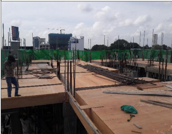
Figure 3.3- 7 th floor slab formwork
