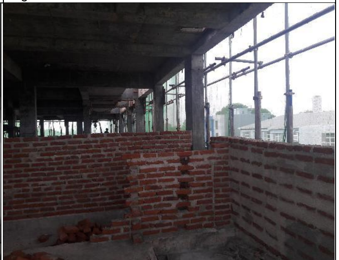
Figure 3.12-5 th floor Brick works
