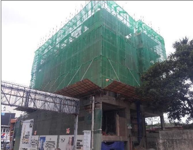
Figure 3.1- Front view from base line
