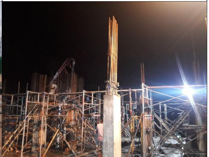
Figure 3.4- 6 th floor column casting
