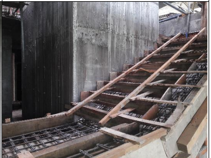
Figure 3.10-staircase 4 th to 5 th .
