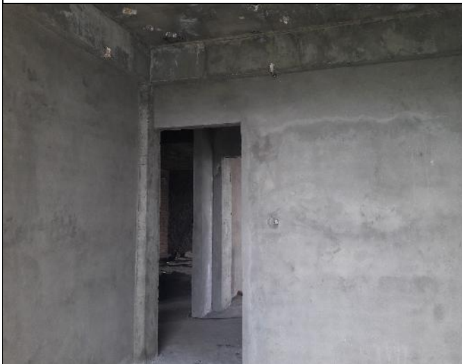
Figure 3.9- 3 rd floor plastering
