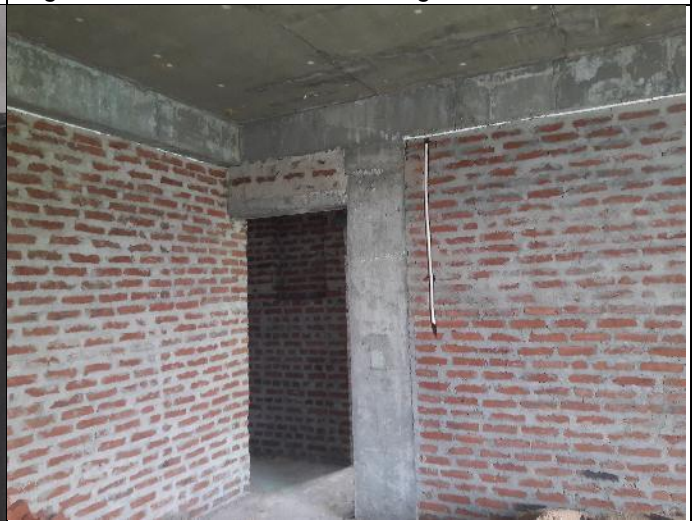
Figure 3.6-4 th floor Brickworks
