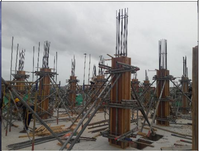
Figure 3.4- 7 th floor column formwork
