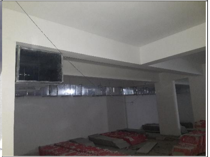
Figure 3.10-basement fresh air service
