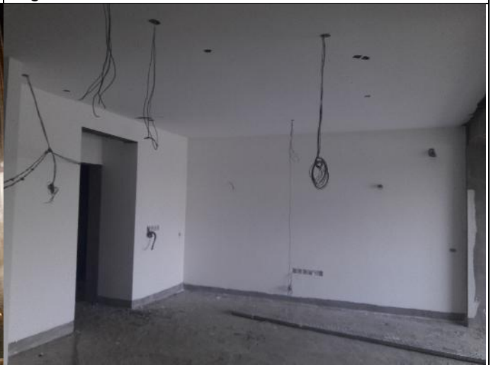
Figure 3.6-3 d floor wall putty
