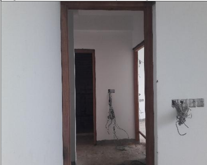
Figure 3.11- 2 nd floor timber frame
