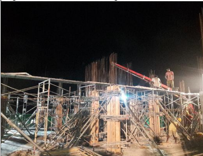
Figure 3.5-7 th floor column casting
