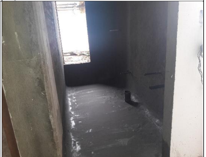
Figure 3.12-2 nd floor waterproofing
