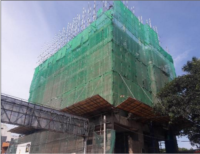
Figure 3.1- Front view from base line
