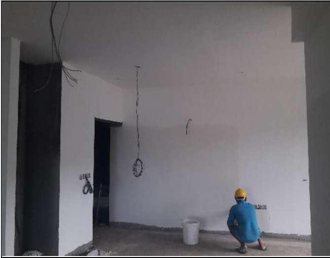
Figure 3.7- 4 th floor wall putty
