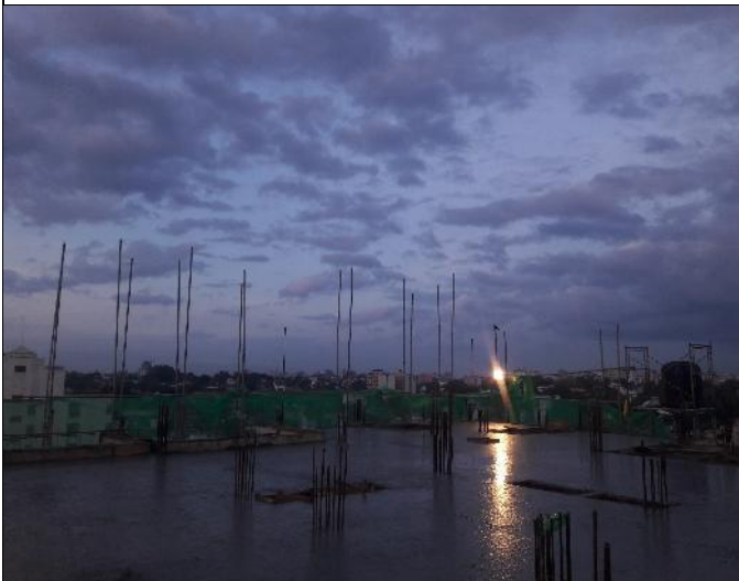
Figure 3.3- 7 th floor slab casting
