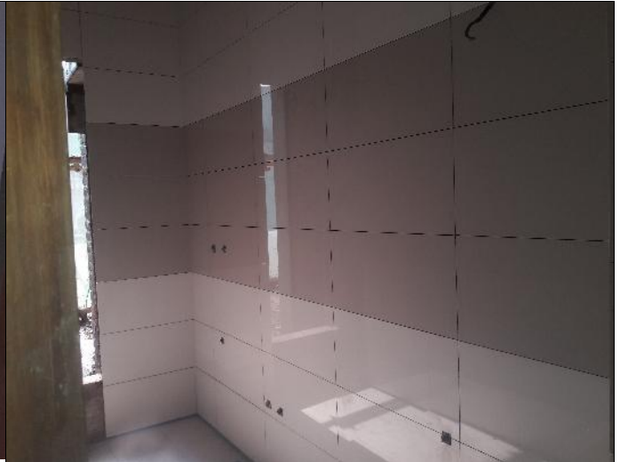
Figure 3.8 – 2 nd floor bathroom tiling
