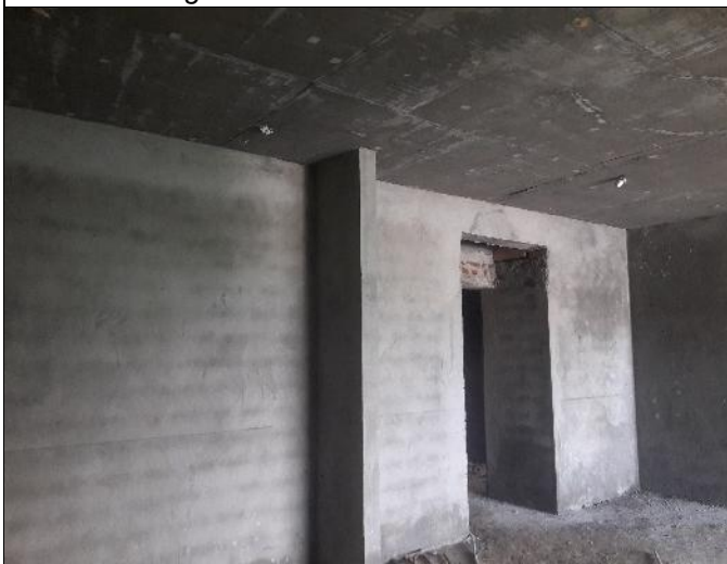
Figure 3.5 - 6 th floor plastering
