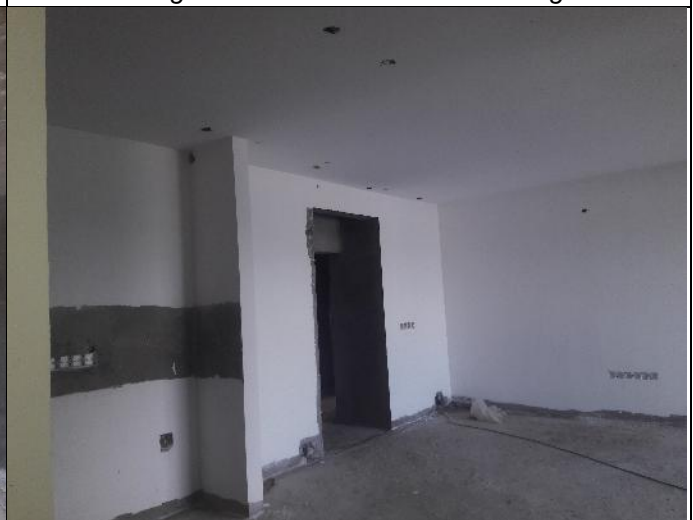
Figure 3.6 - 5 th floor wall putty
