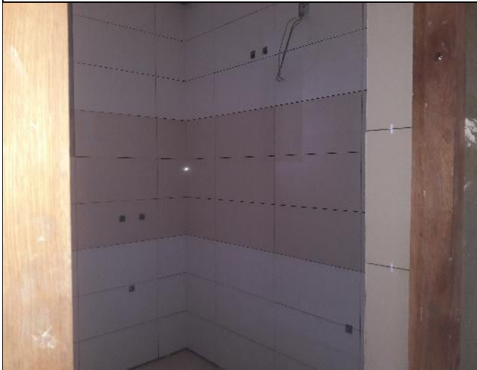
Figure 3.9- 2 nd floor bathroom tiling
