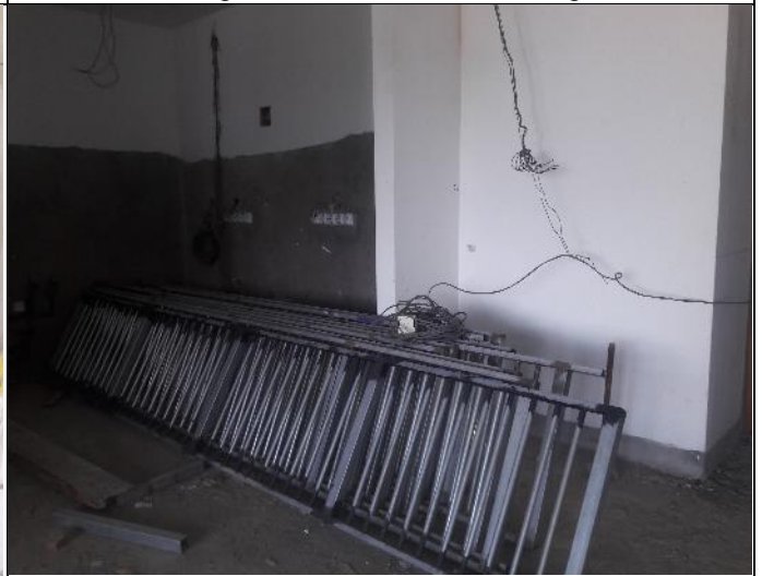
Figure 3.12-handrail fabrication
