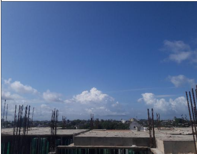
Figure 3.3- 9 th floor slab formwork
