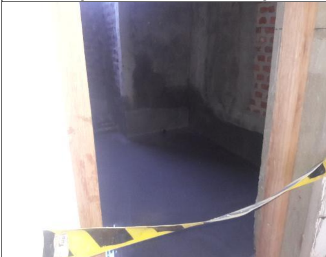
Figure 3.11- 3 rd floor bathroom waterproofing
