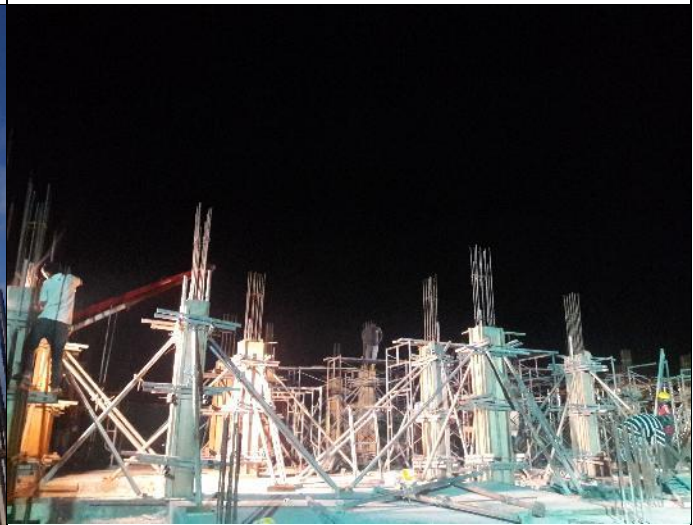
Figure 3.4- 8 th floor column Casting
