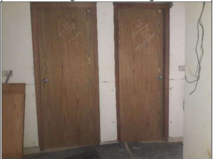
Figure 3.12-3 rd floor internal doors
