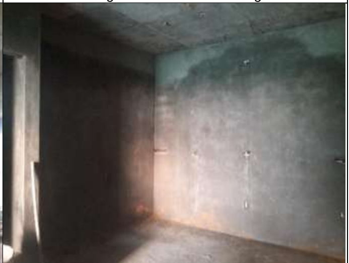
Figure 3.6 8 h floor plastering
