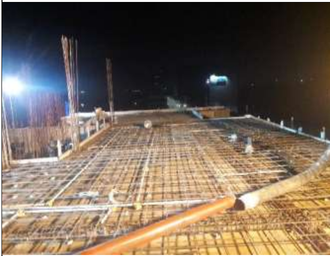
Figure 3.3- roof slab r/f& f/w
