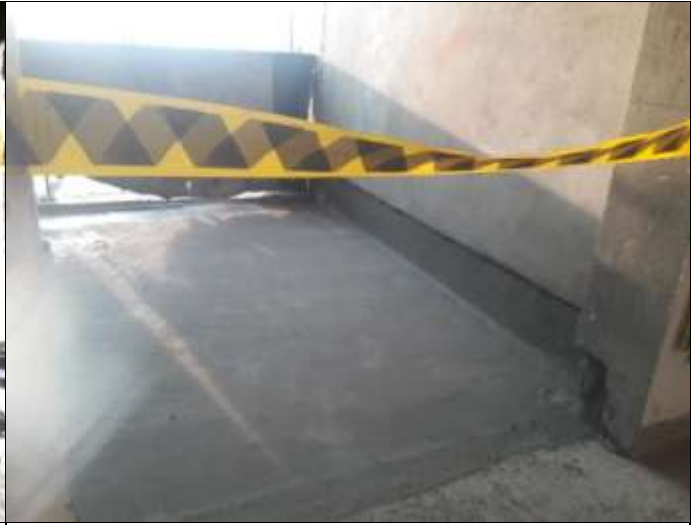
Figure 3.8 – 5 th floor balcony waterproofing
