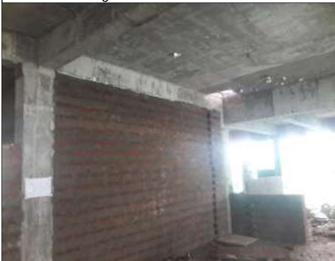
Figure 3.5-8 th floor brick works
