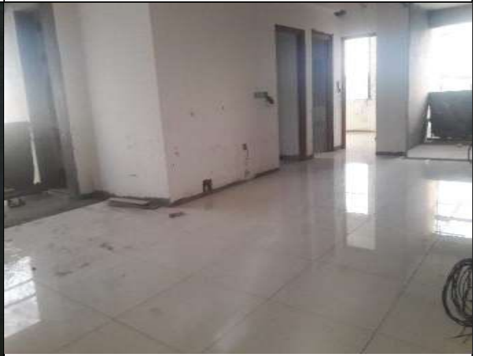
Figure 3.10-4 th floor tiling
