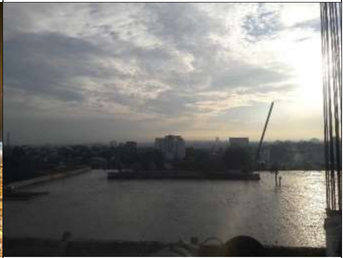
Figure 3.4- roof slab casting
