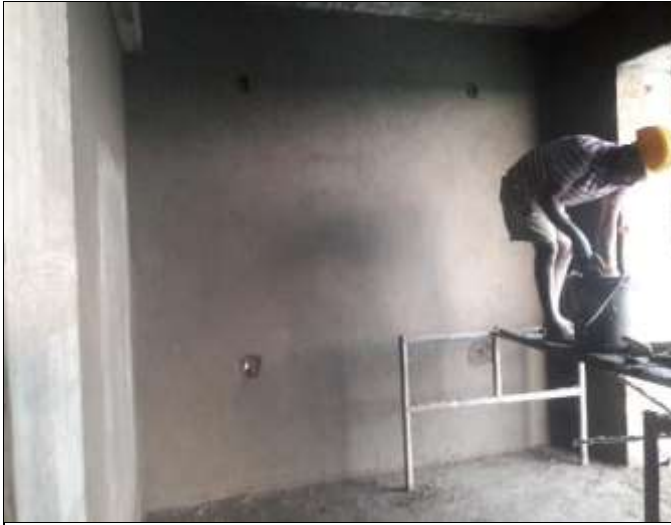
Figure 3.7- 7 th floor plastering
