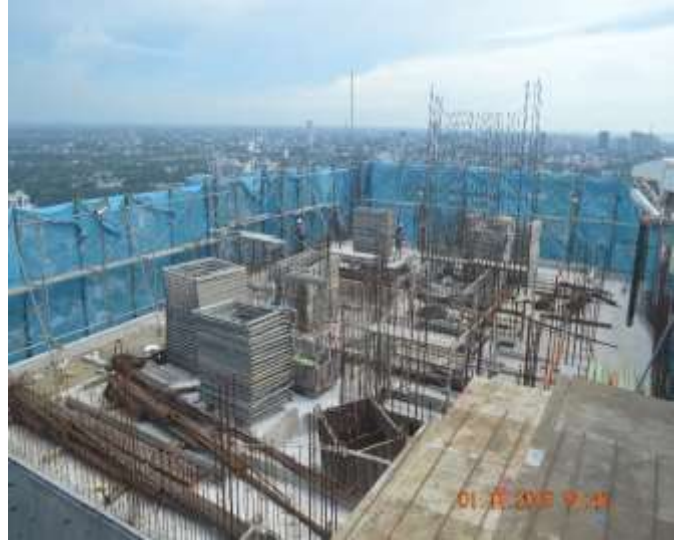
Figure 3.2 – Formwork for slab 30 th floor
