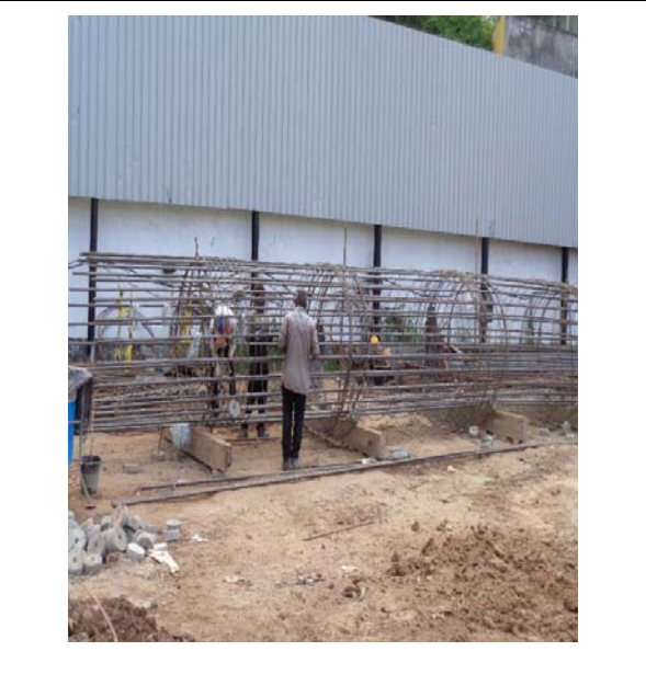
Figure 4 – Pile reinforcement cage fabrication work
