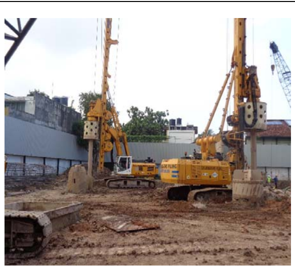
Figure 2– Pile Boring in Progress
