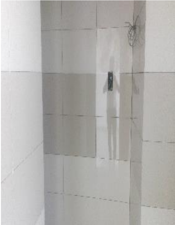
Bathroom Tiling work
