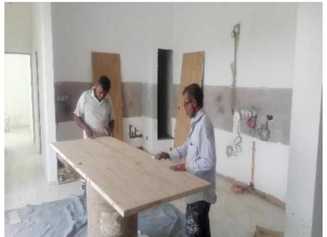
Door sash finishing Works
