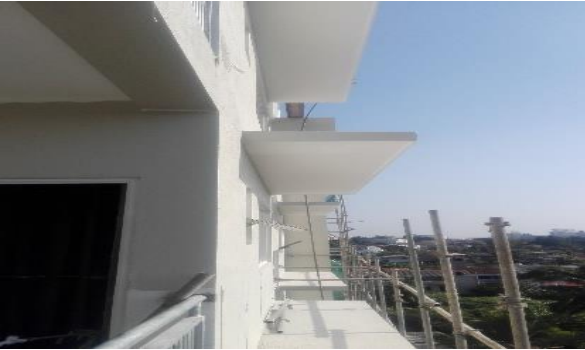
External Painting Work
