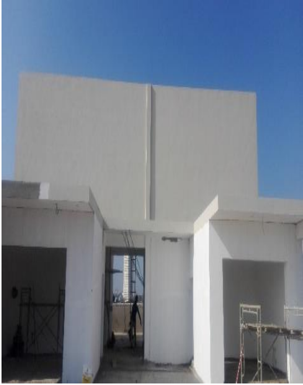
Plastering and painting Work at Roof Terrace
