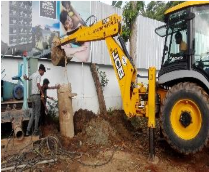
Casing installed
