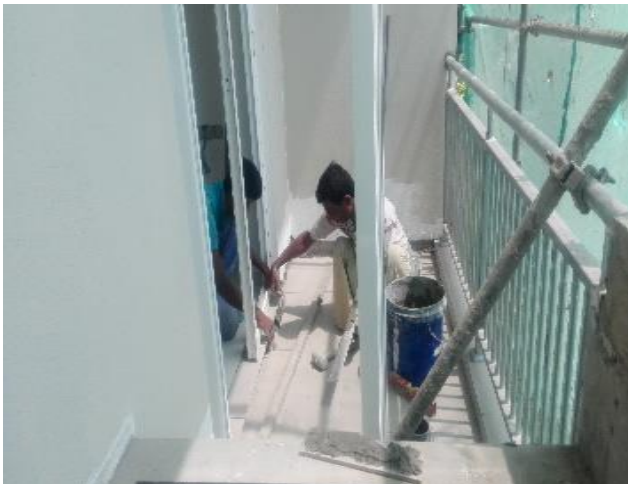
Floor Tiling work
