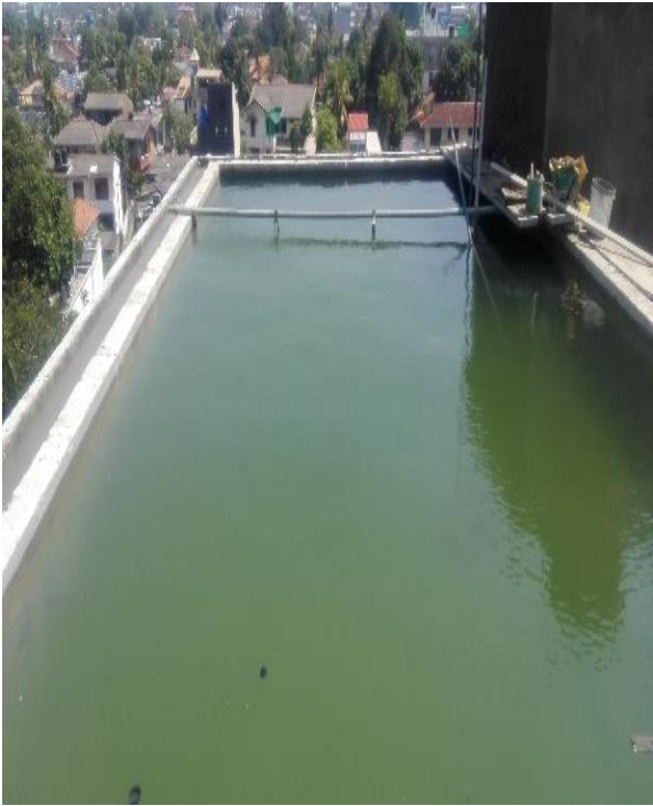
Swimming Pool work in progress
