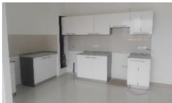
Fixing Pantry cupboards
