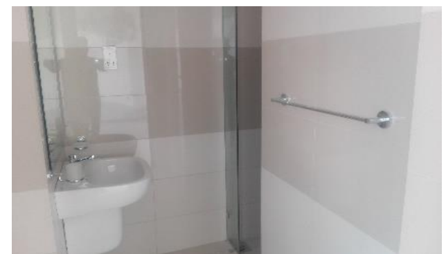
Figure 1.6 : Bathroom Tiling work
