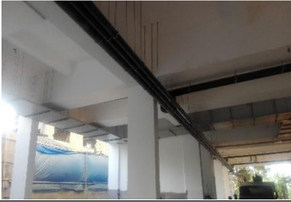
Figure 1.7 :Ground Floor Plumbing work
