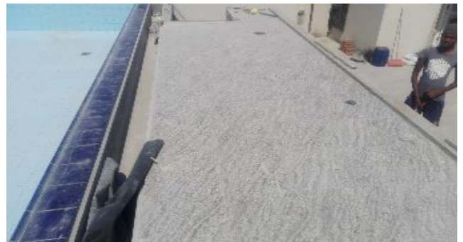
Figure 1.12 : Pool Deck tiling
