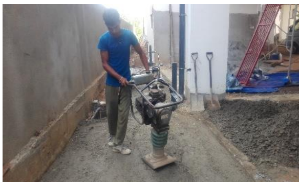
Ground Floor Compaction
