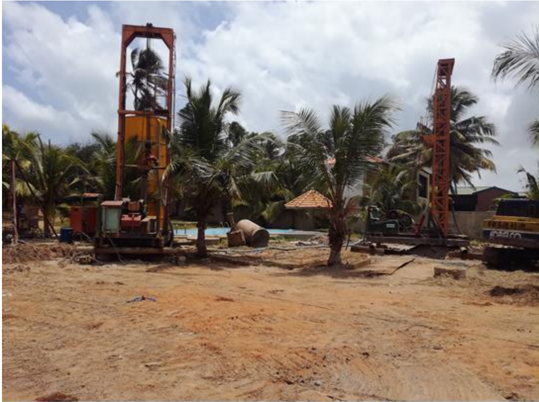
5th & 6th Pile boring work
