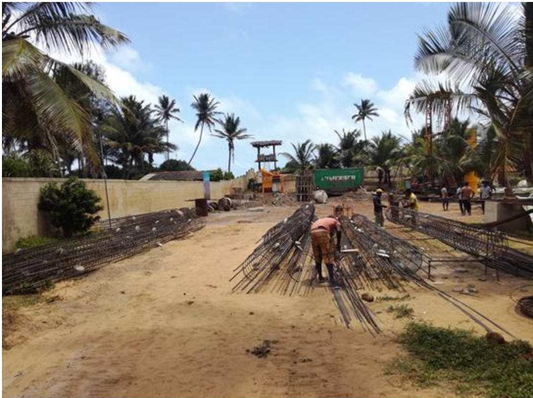
Pile Reinforcement work on Progress
