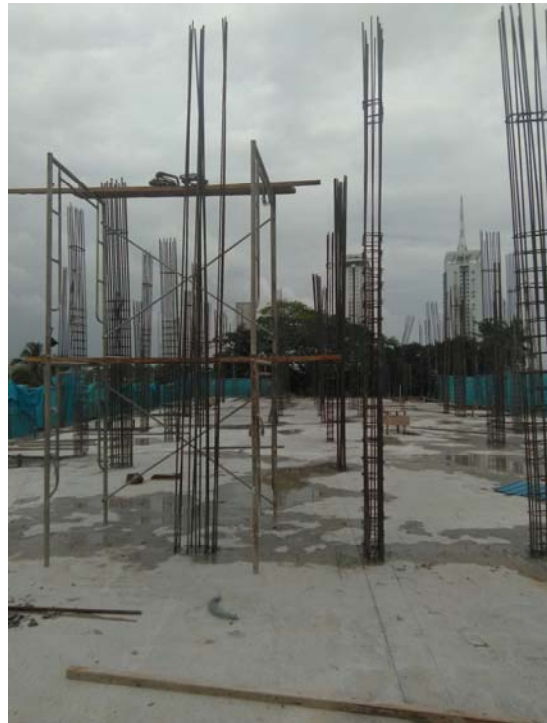
2 nd Floor Slab After Concreting (Zone B)
