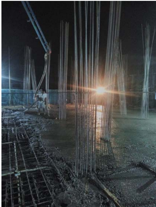
2 nd Floor Slab Concreting (Zone B)
