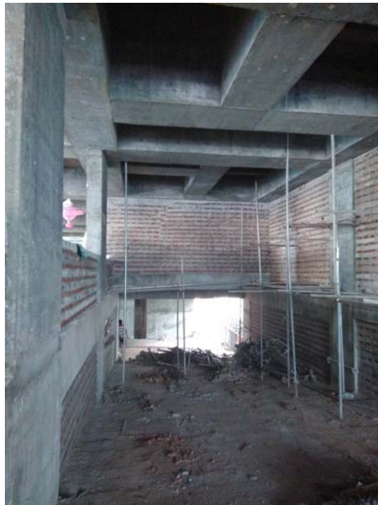
Brick Work at 2 nd Floor
