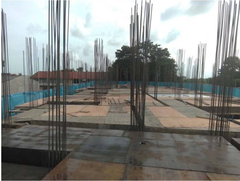
4 th Floor Slab (Zone A)
