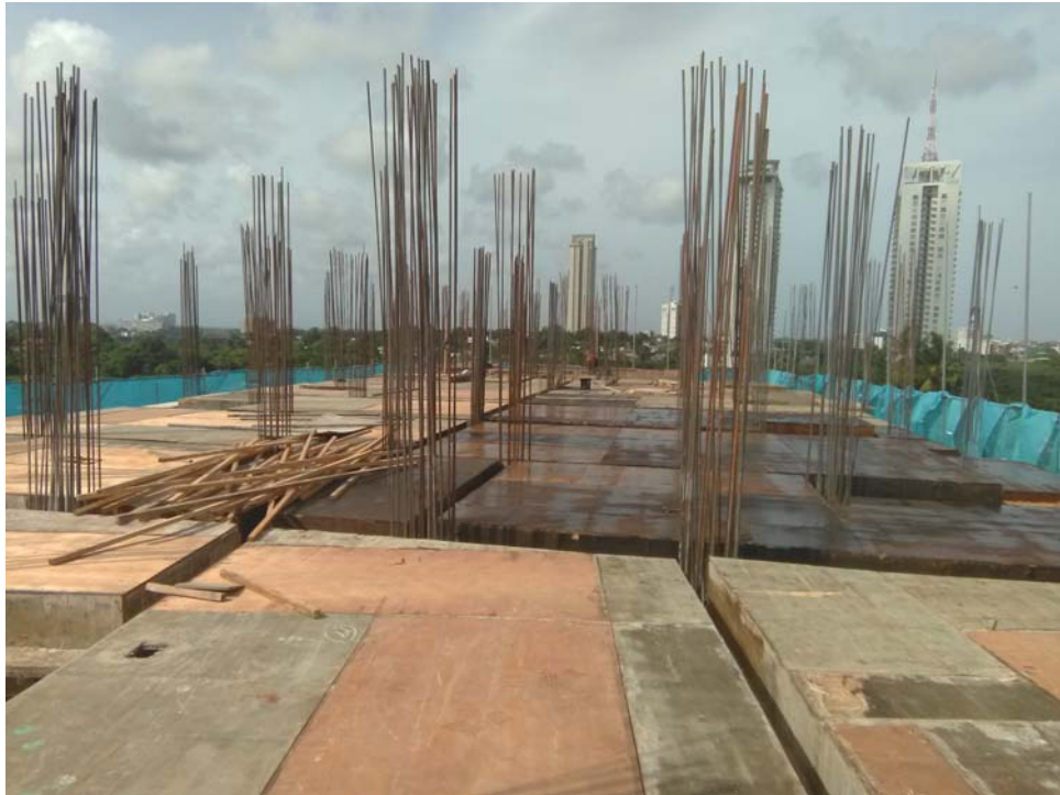
4 th Floor Slab (Zone B)
