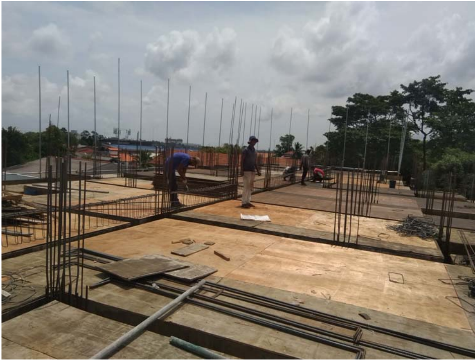
Form Work and Reinforcement Work for 5 th Floor Slab (Zone A)
