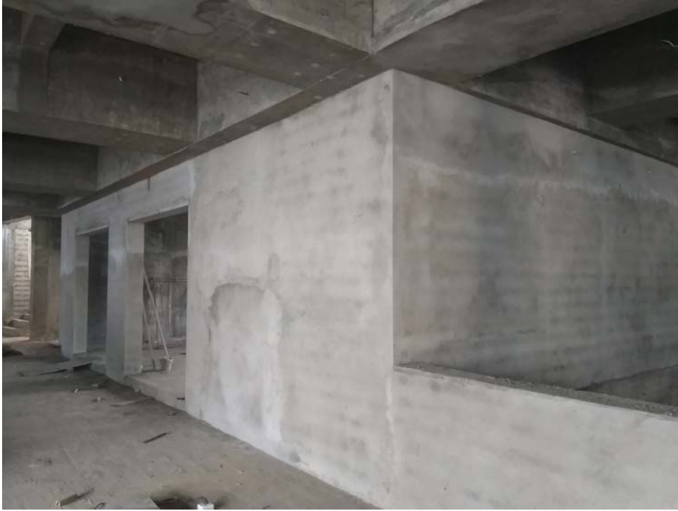
Plastering Work at 1 st Floor
