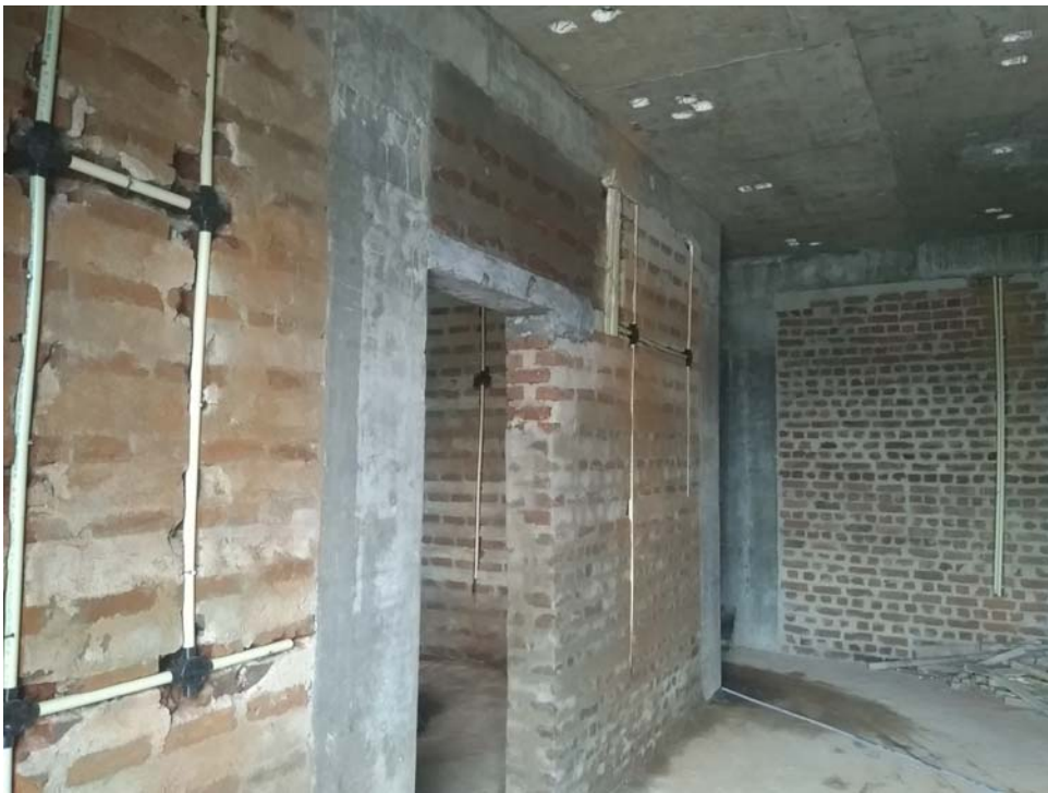
Brick Work at 2 nd Floor
