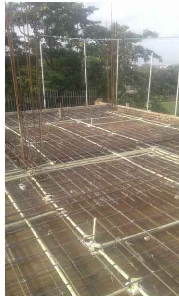
Reinforcement Work for 6 th Floor Slab
