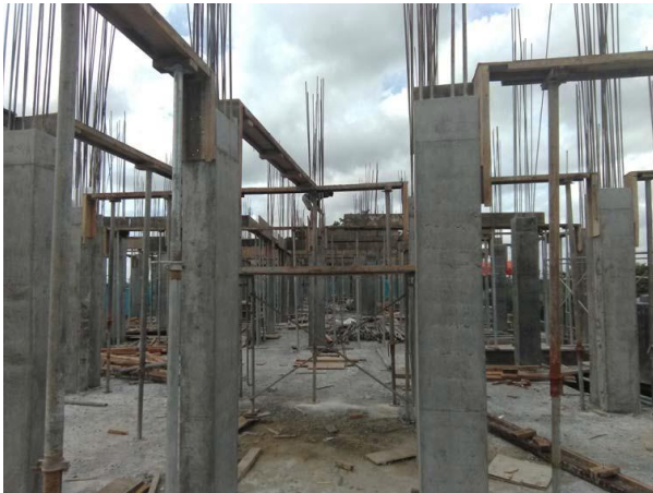
Form Work for 6 th Floor Slab
