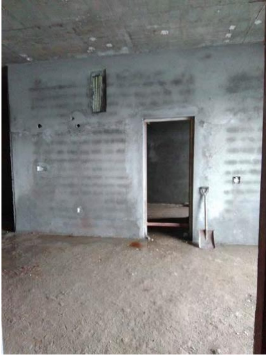
Wall Plastering at 2 nd Floor
