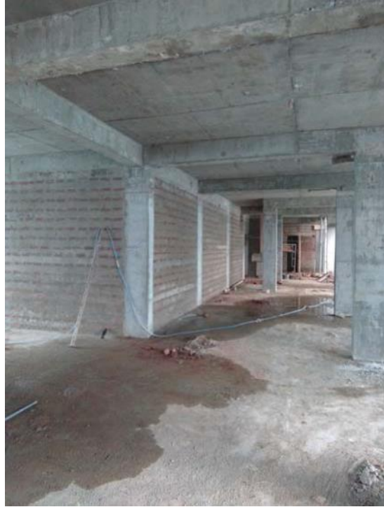
Brick Work at 3rd Floor
