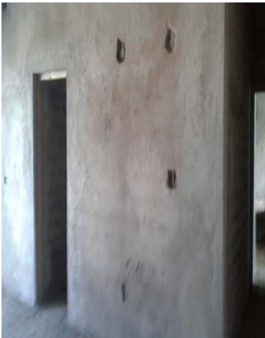
Wall plastering at 4 th floor
