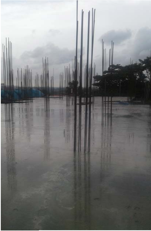
7 th Floor Slab Casted
