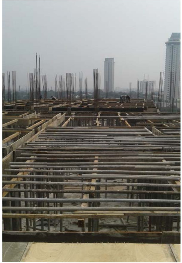
Form Work - Roof slab
