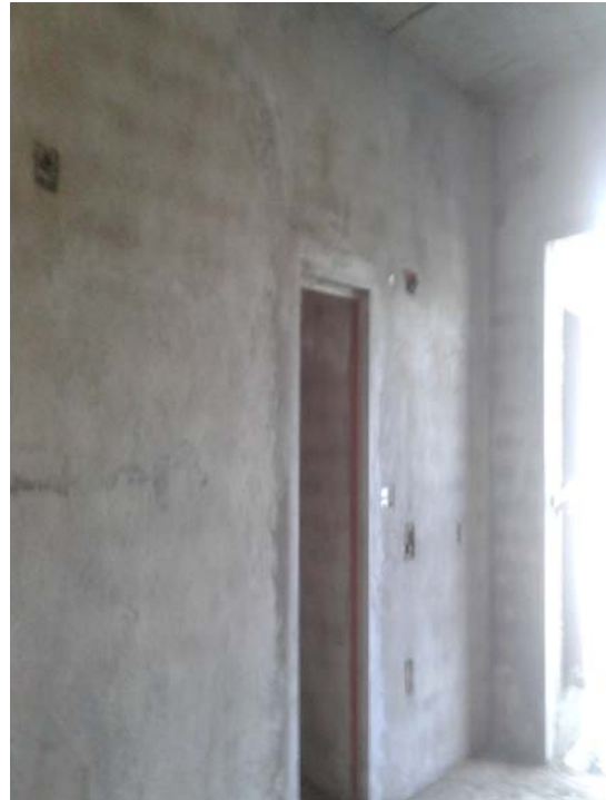
Wall Plastering at 3 rd Floor
