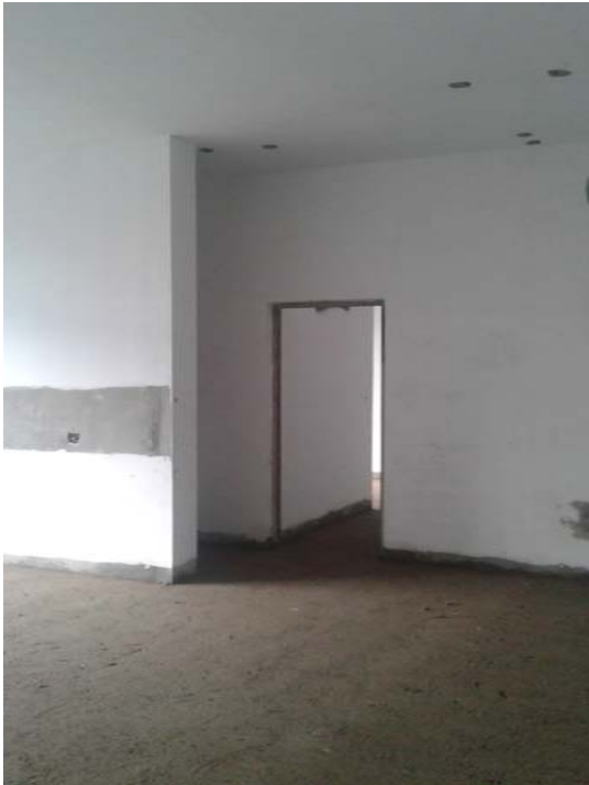
Putty Application at 2 nd Floor
