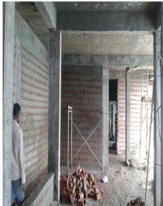
Brick work at 5 th Floor
