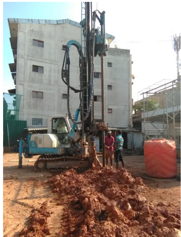
Installation of H iron for Shoring
