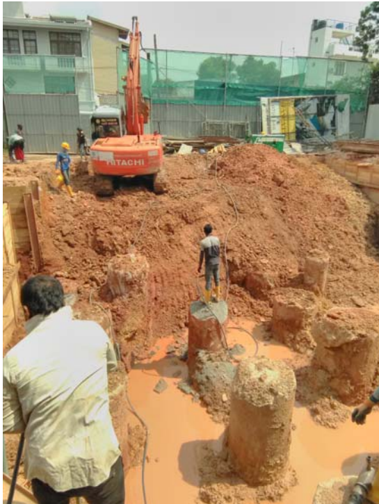
Excavation for Basement Floor
