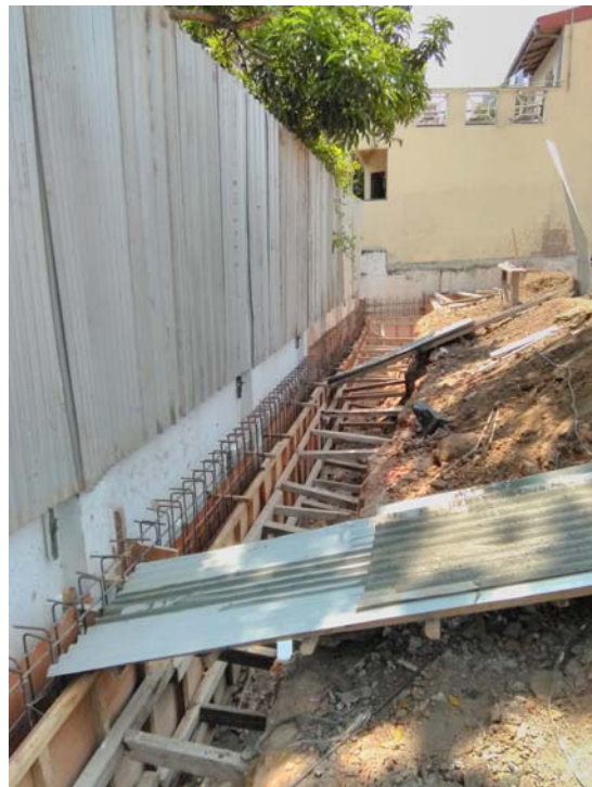
Ready for Boundary Wall Concreting
