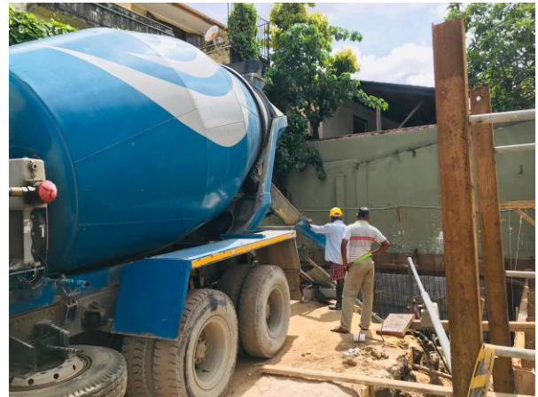
Water Sump Base Concreting
