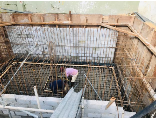
Water Sump Base R/F Work
