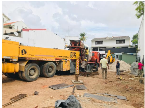
Pile Caps & Ground Beams Concreting – Part I
