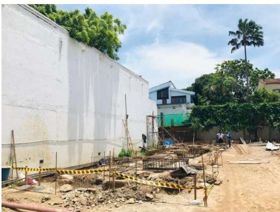
Pile Caps & Ground Beams R/F Work on Progress
