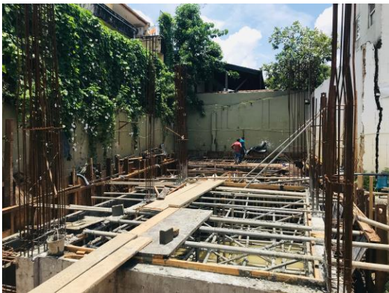
Structural Works on Progress around Water Sump
