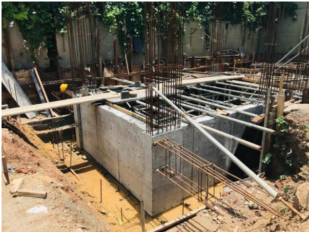
Car Lift Base & Walls Concreting Completed
