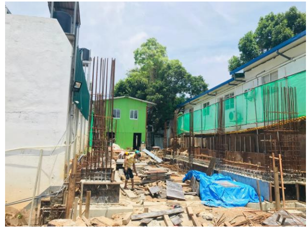
Retaining Walls & Columns on Progress
