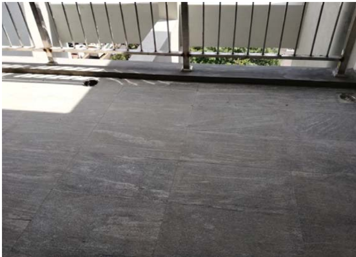
Balcony work completed
