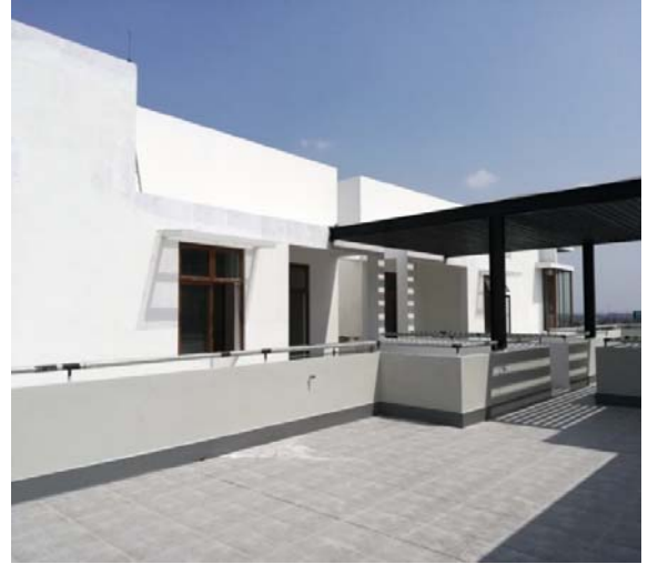
Roof terrace view
