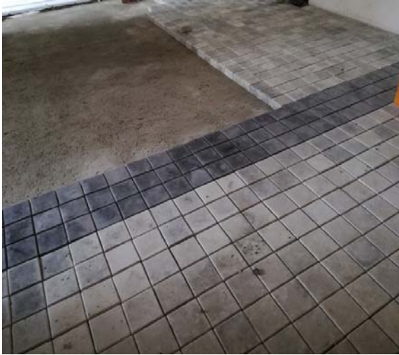
Paving work on progress
