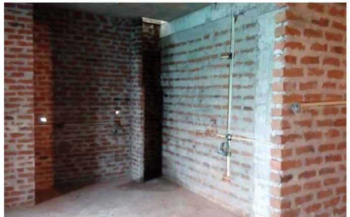
5 th floor Brick work on progress
