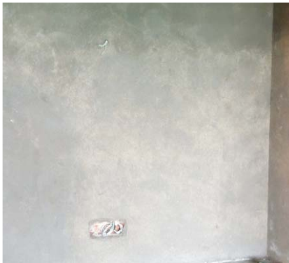
Plastering on progress
