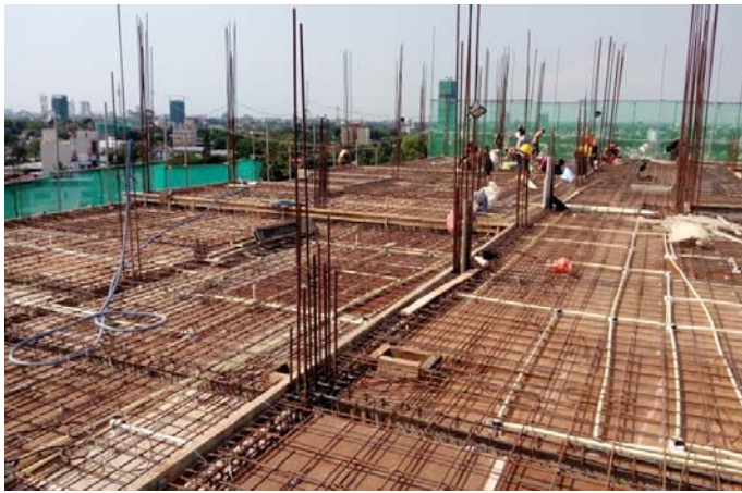
8 th floor work on progress
