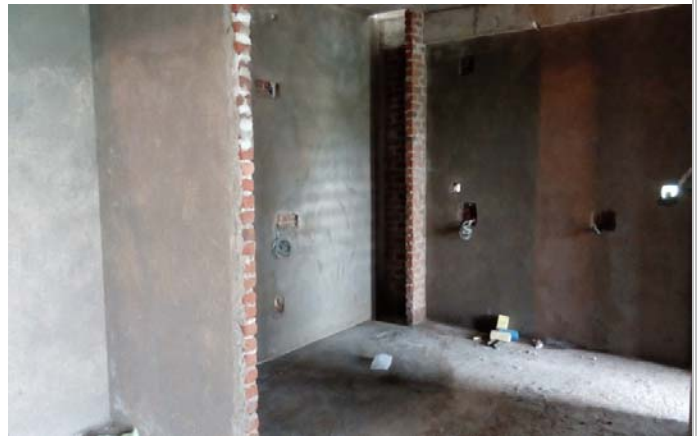
Wiring work on progress
