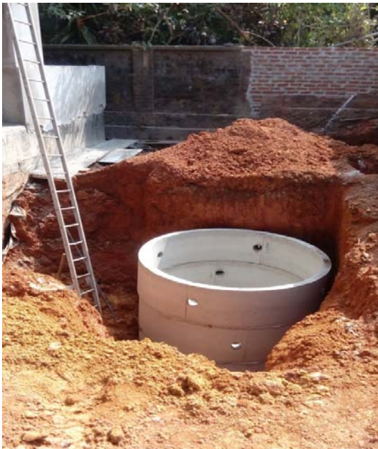
Septic & soakage pit work on progress
