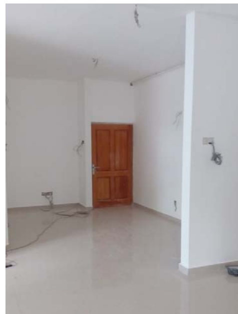
Internal painting on progress
