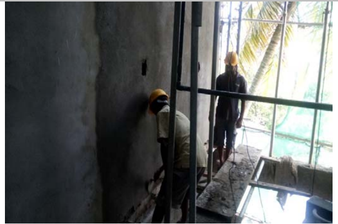
Wall Plastering Work at 4 th Floor
