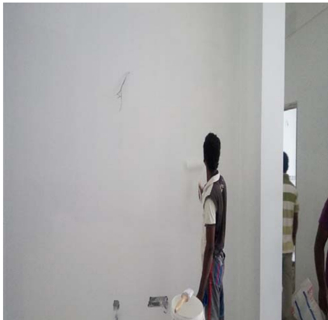
Painting Work at 1 st Floor
