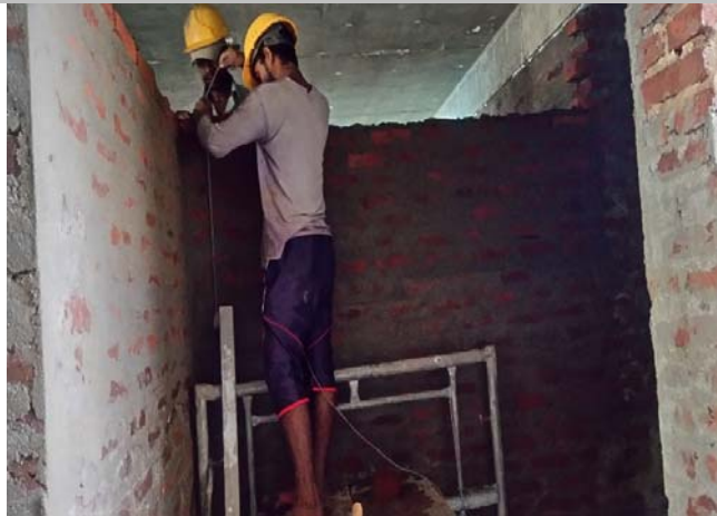
Brick Work at 5 th Floor
