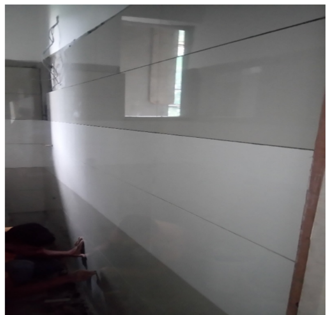
Toilet wall tilling work at 1 st Floor
