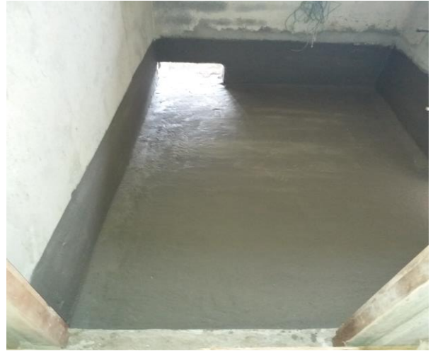
8 th Floor Water Proofing Work
