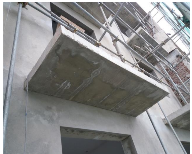
External Plaster work
