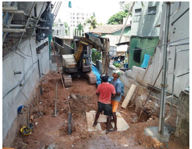
Sewerage Treatment Plant Work
