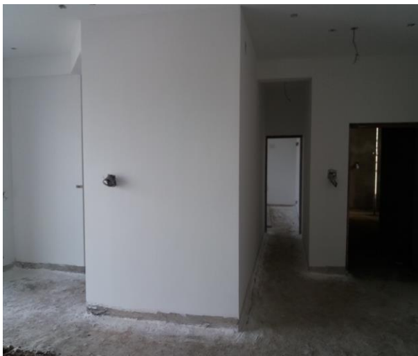
8 th Floor Painting Work
