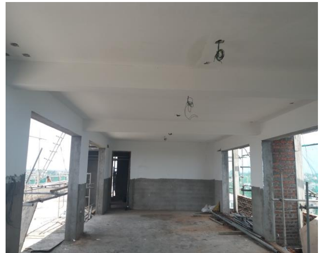
Roof Terrace Painting Work
