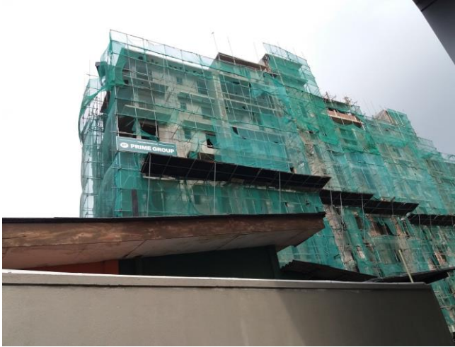
External Plaster work
