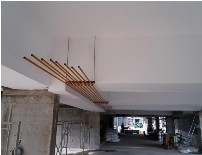
Ground Floor Gas Work
