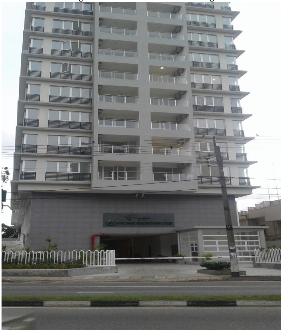
Figure 02 - Front View of the Building
