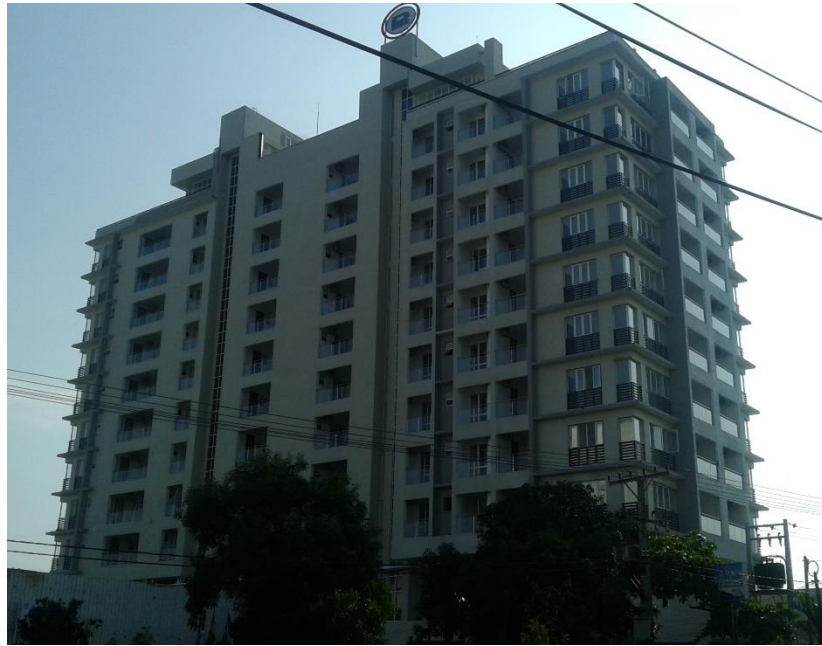
Figure 01 – Side View of the Building
